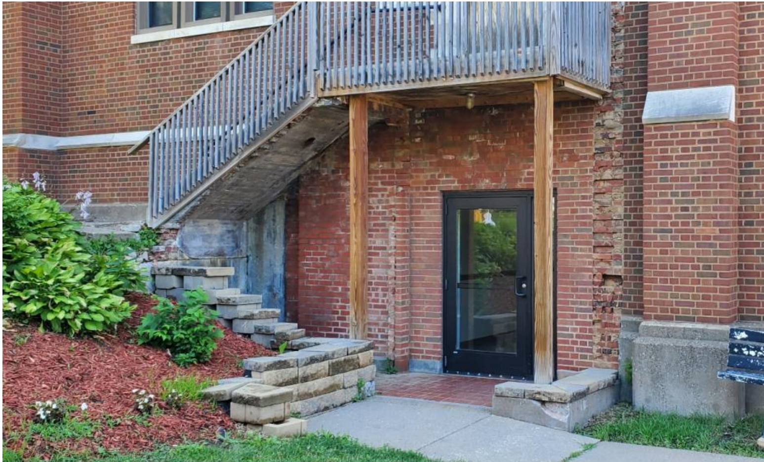
West Entrance: Evidence of Brick Vestibule
