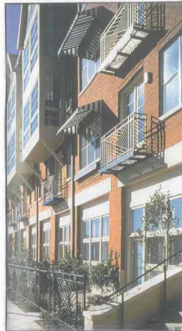
CPTED principles in practice. Ornamental fencing denies access and creates clear boundaries giving the residents a stronger sense of territoriality. Finally, the many windows and balconies provide for natural surveillance.
