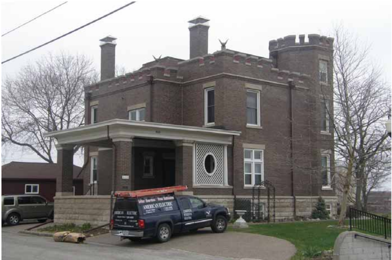
Photograph 82-02494-003 - House, looking southeast (April 2015)
