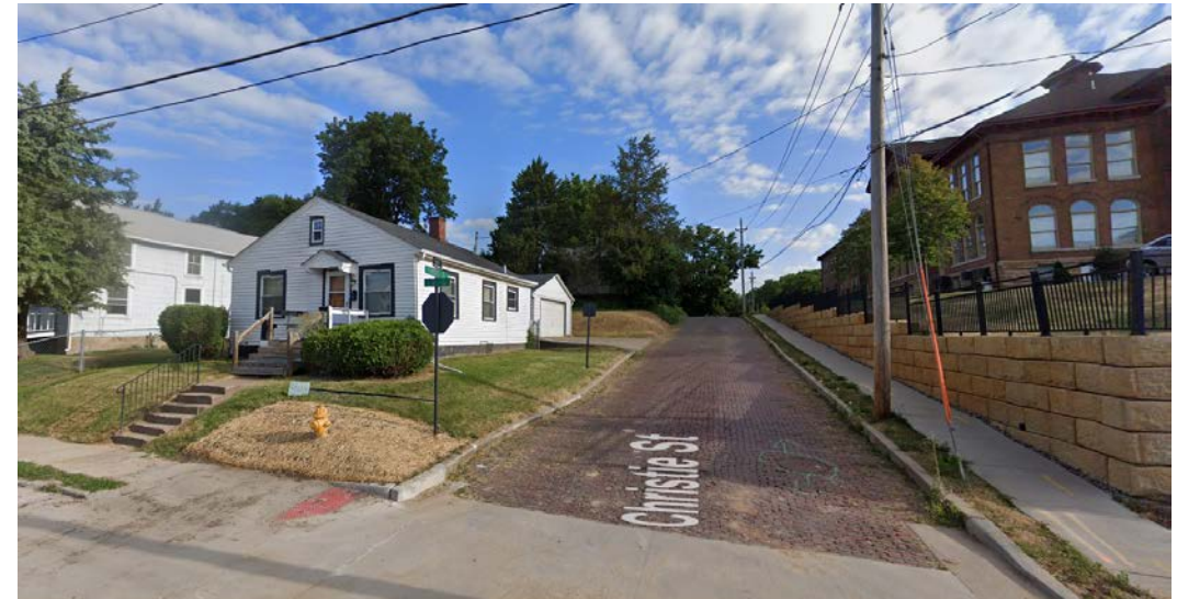
View From East 12 th Street - Facing North
