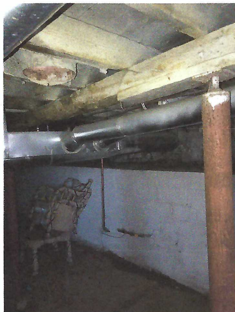
6x4 wood beam and support column.
