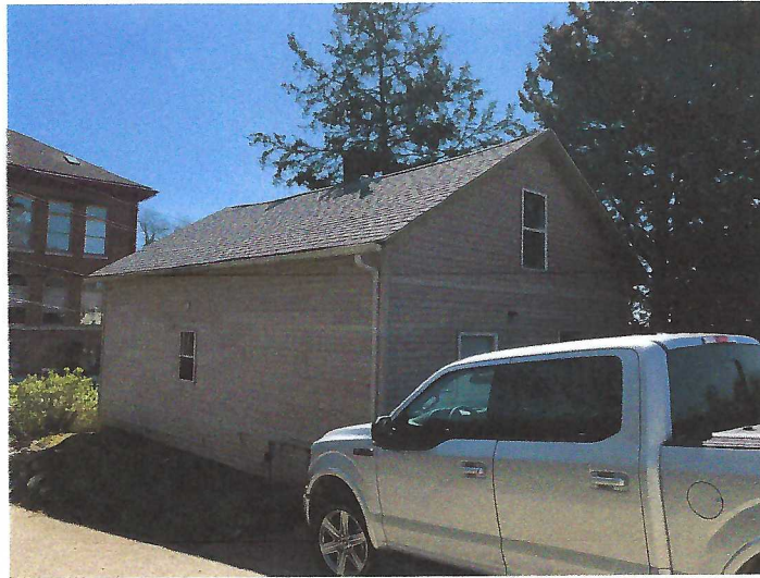
View of the residence facing southeast.
