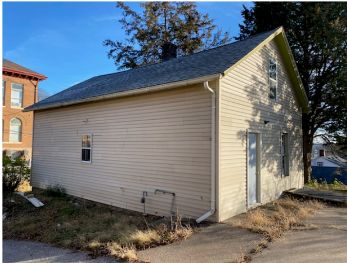
Northwest Elevation-View From Alley
