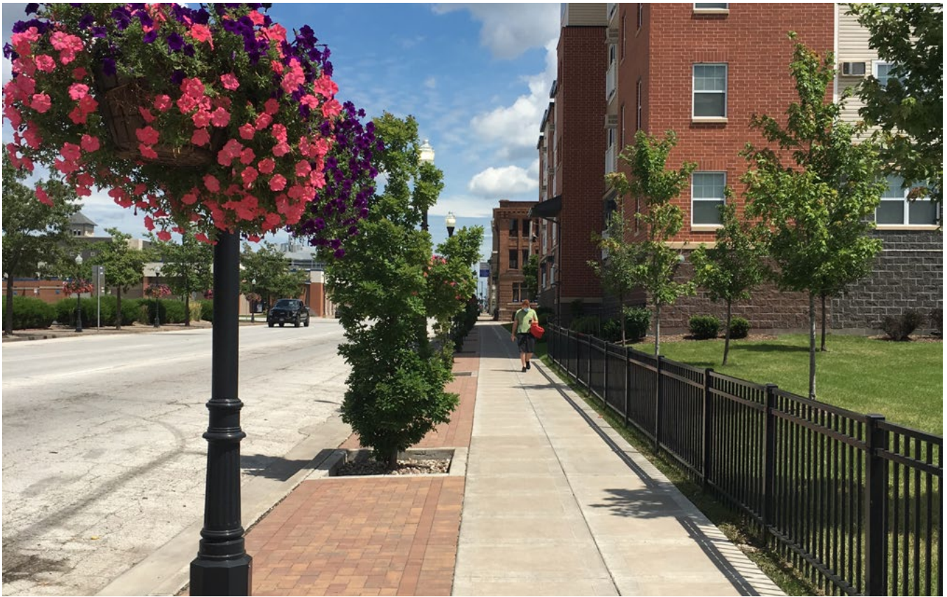
Newly constructed streetscape on 3rd Street
