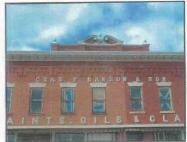
Detail: Ranzow Paint Company Building constructed in 1875.
