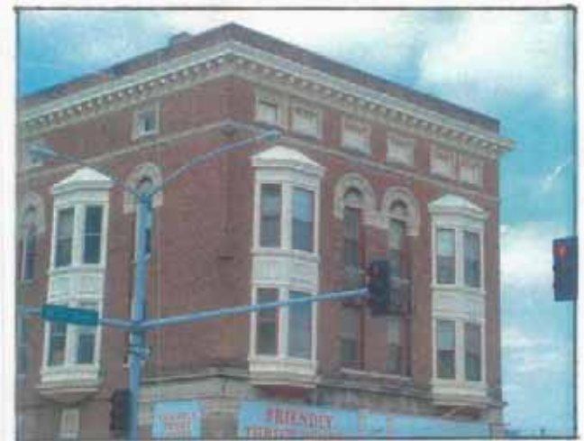
Detail: Ficke Building constructed c. 1900.
