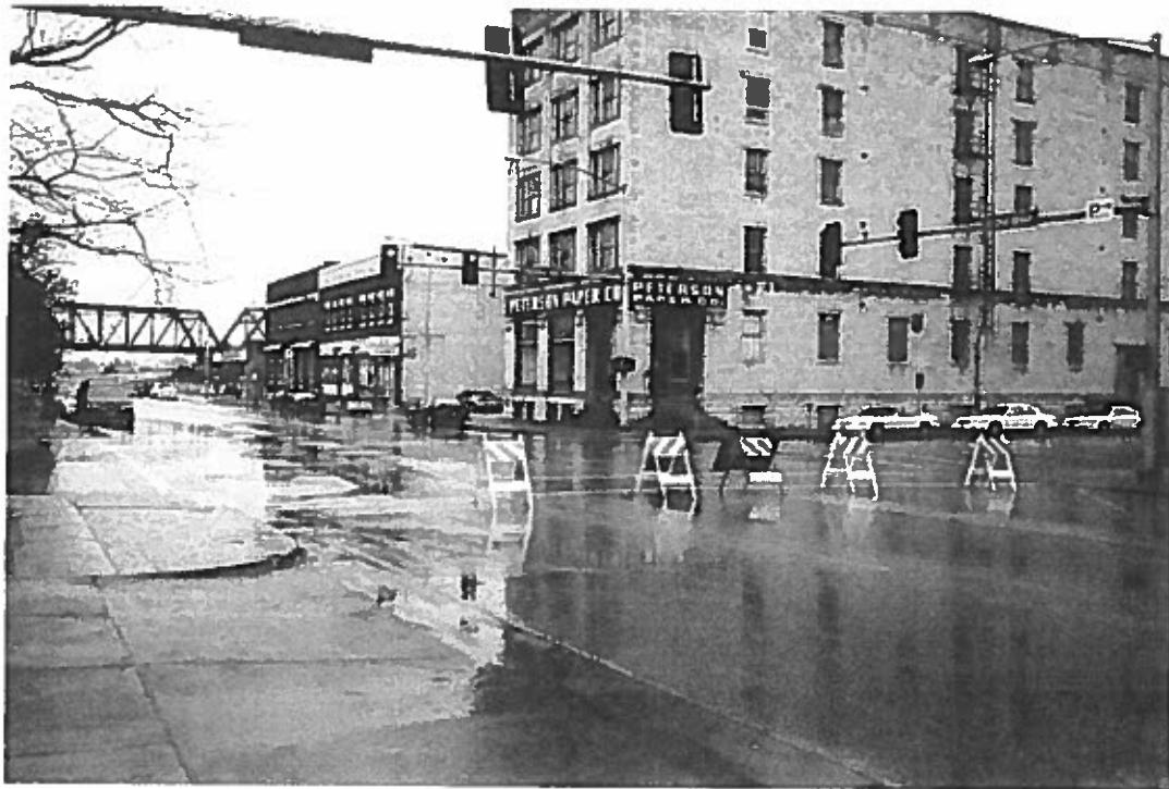
View of Iowa Bearing Co., Inc. within the context of its streetscape (looking east along E. 2nd Street from Pershing.)
