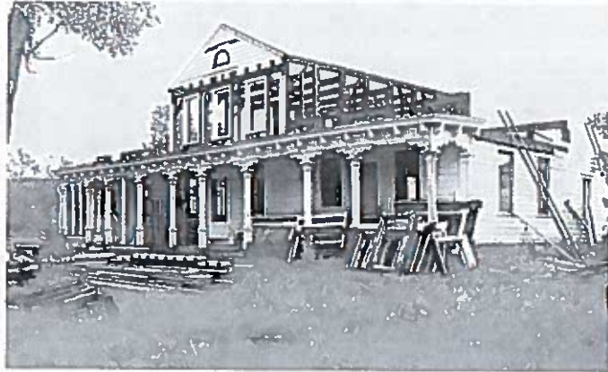
Dismantling of Bruchmann residence, May 2000
