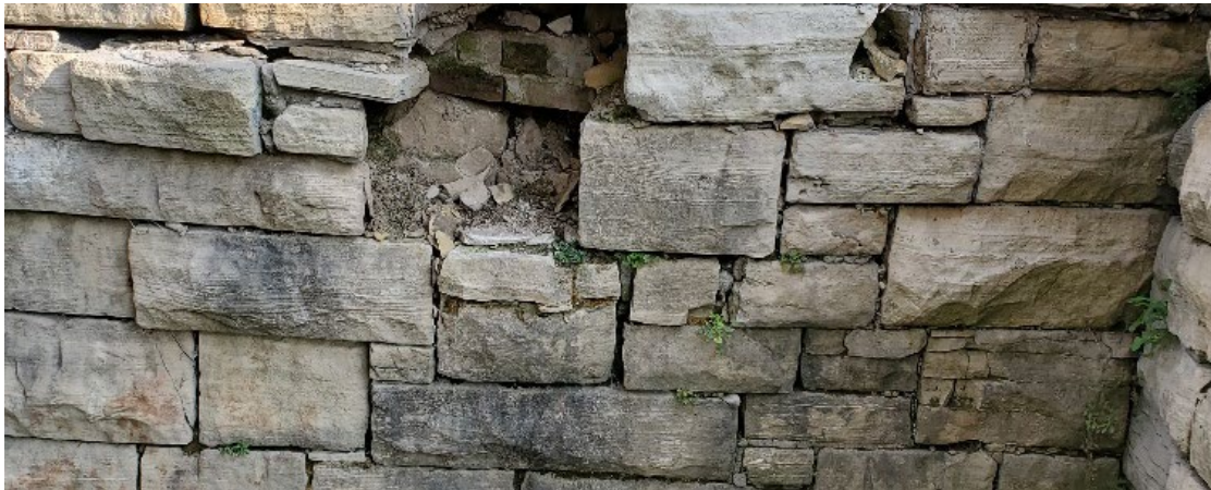
Failed Retaining Wall at E 6 th Street & Iowa Street
