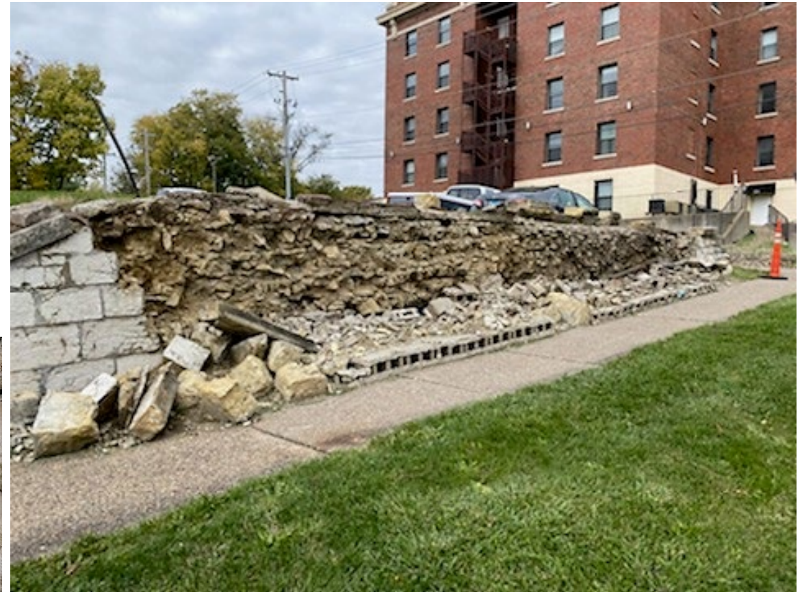
Failed Retaining Wall at E 6 th Street & Iowa Street
