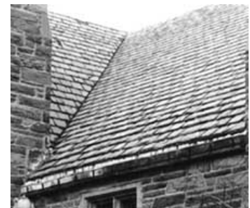
Valleys are formed at the internal angle of two roofing slopes. Flashing is often placed under the slate to increase moisture protection at this vulnerable joint. Photo: Jeffrey S. Levine.
