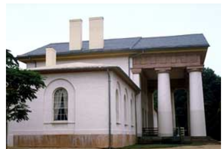
Although slate replacement roofs are expensive, the superiority of materials and craftsmanship will give
