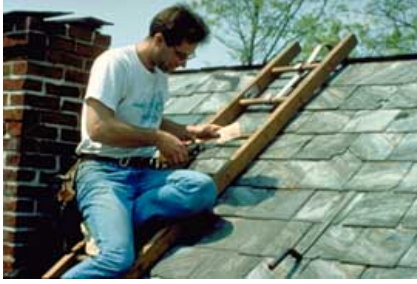
After removing the deteriorated slate and sliding the new slate into place, it is secured with a copper nail. A copper bib (shown here) is formed to protect the newly created nail hole. Finally, a slate hammer is used to push the bib in place over the nail head. Photo: Jeffrey S. Levine.
