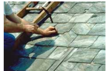
Slate roof repair. Photo: Jeffrey S. Levine.
