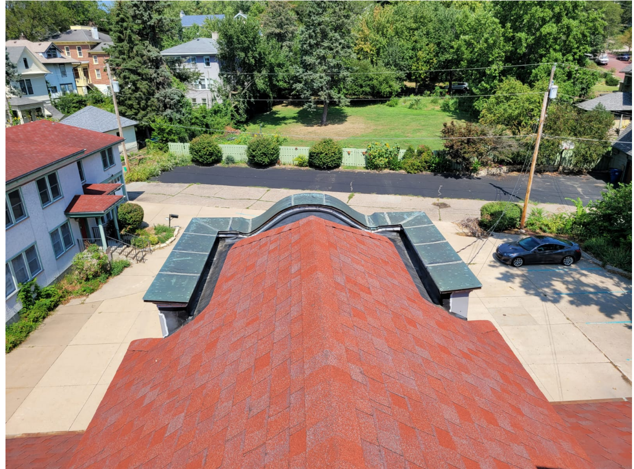
Existing (Non-original): Three Tab Asphalt Architectural Shingle Color: Red
