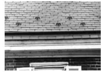
Eave details include snow guards, snow boards, and gutter treatments. Snow guards are generally used in areas where the ice and snow accumulate to avoid dangerous slides from the roof. Photo: Jeffrey S. Levine.
