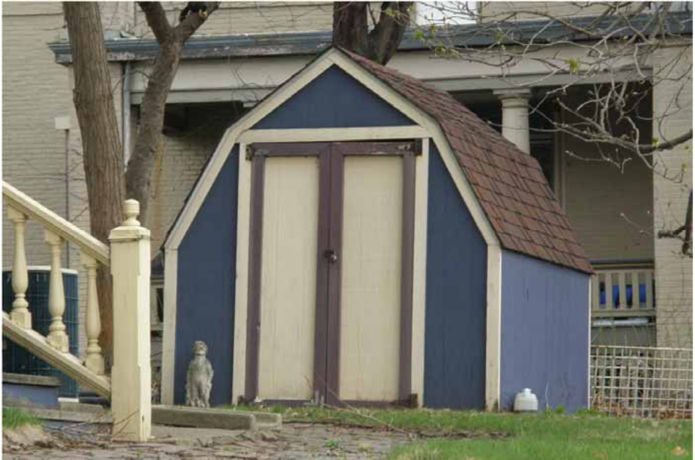
Photograph 82-02670-004 - Outbuilding, looking northeast (April 2015)
