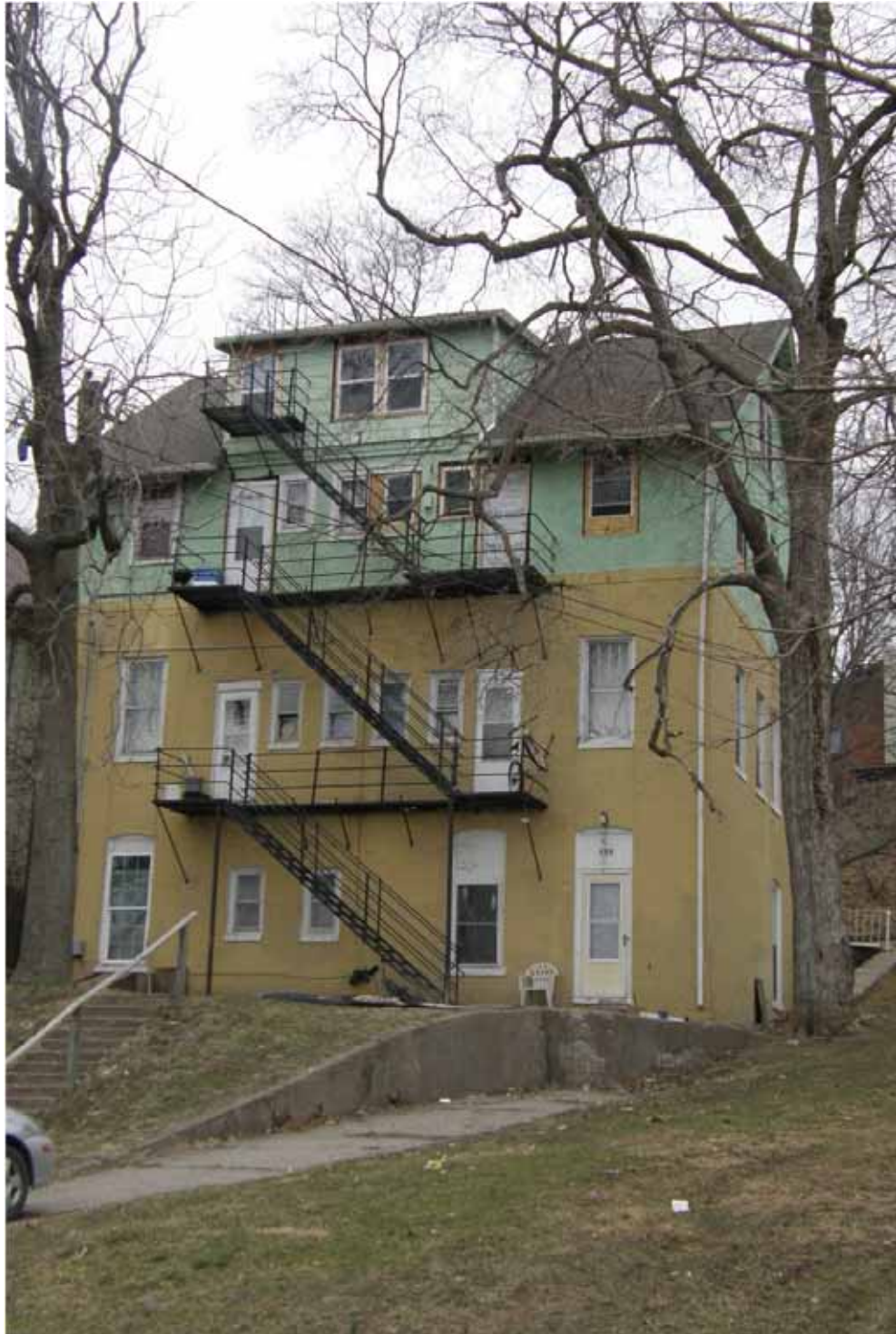
Photograph 82-00552-003 - House, looking northwest (April 2015)
