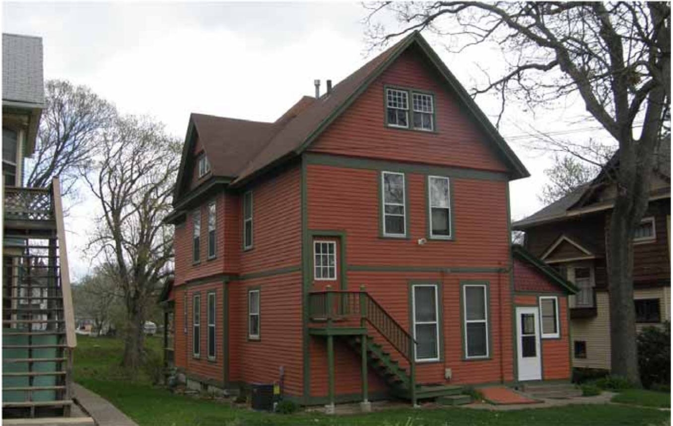
Photograph 82-00680-002 - House, looking northeast (April 2015)
