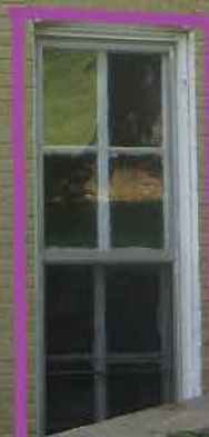
Two Vinyl Double hung windows Custom made to fit opening white ext Alum Clad ext stops.
