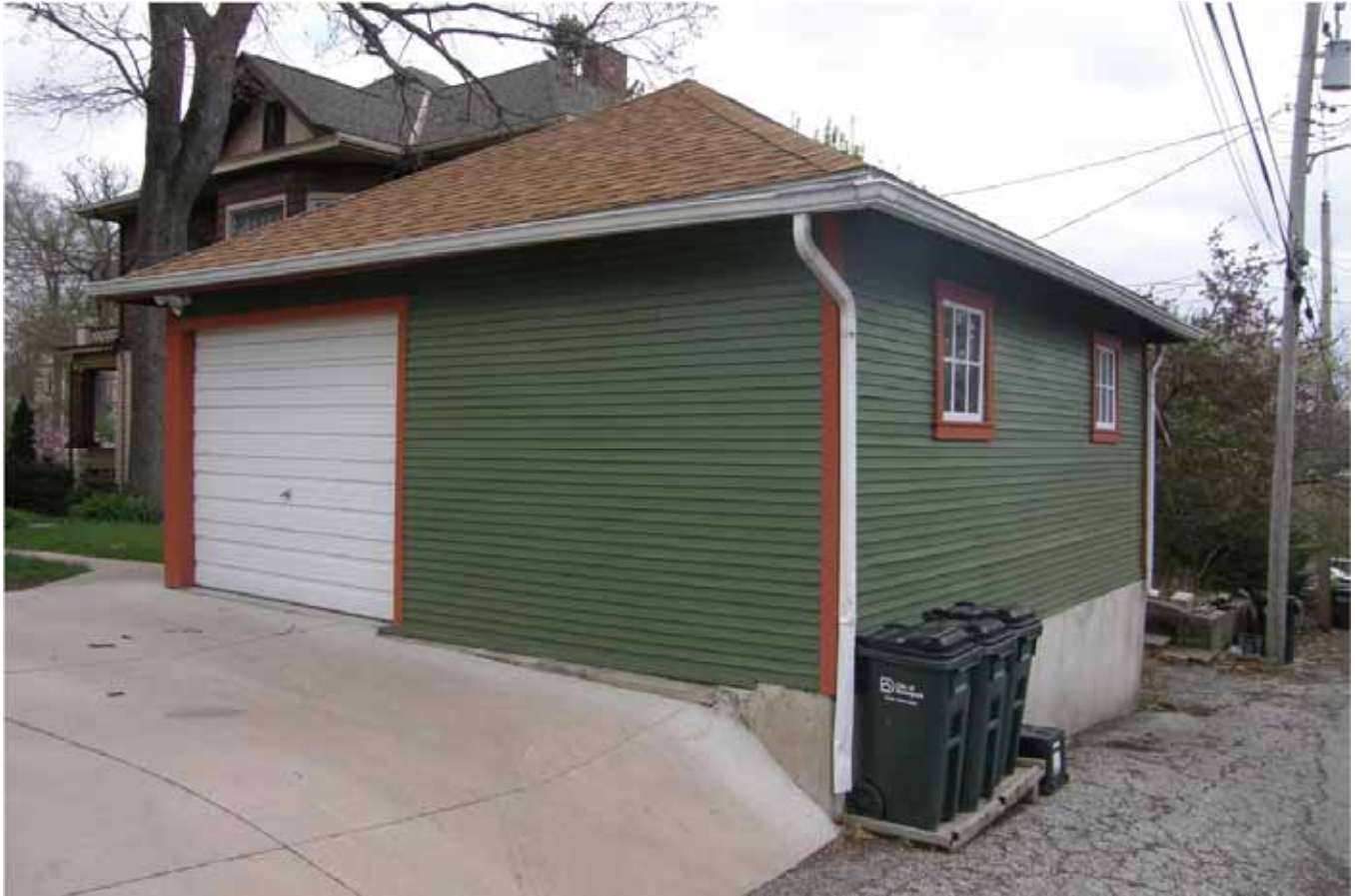
Photograph 82-00680-003 - House, looking northeast (April 2015)
