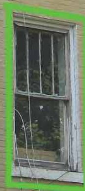
Three Vinyl Double Hung windows white exterior Custom made to fit original opening. Alum Clad exterior stops. There was a fourth that was bricked in.
