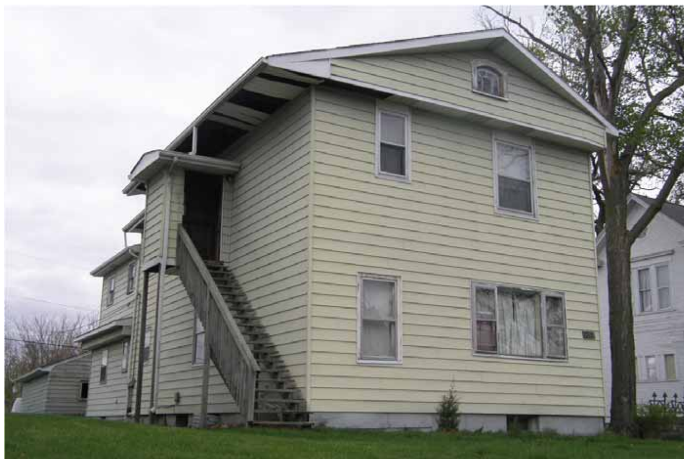
Photograph 82-06970-001 - House, looking northeast (April 2015)
