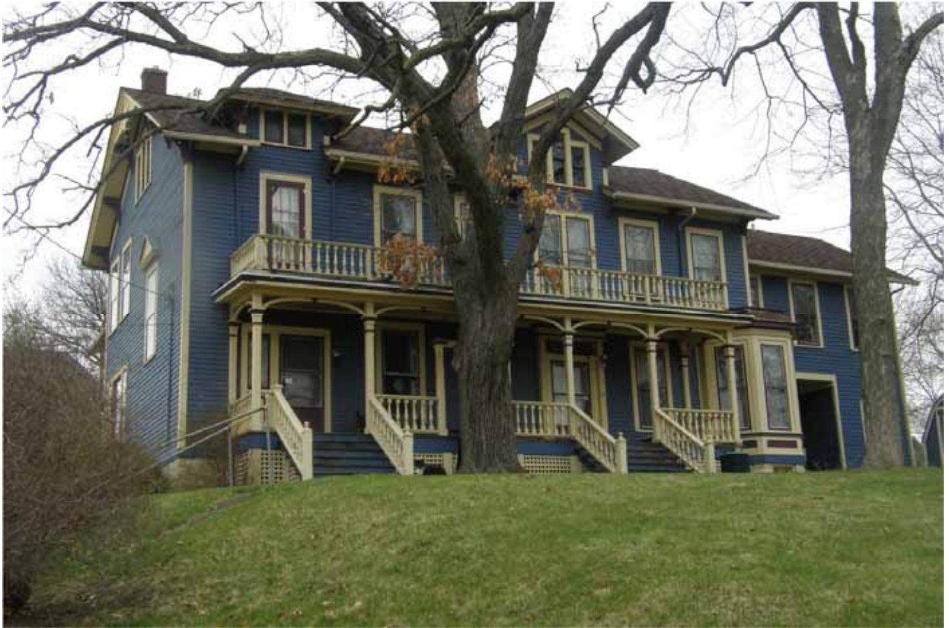
Photograph 82-02670-001 - House, looking northeast (April 2015)
