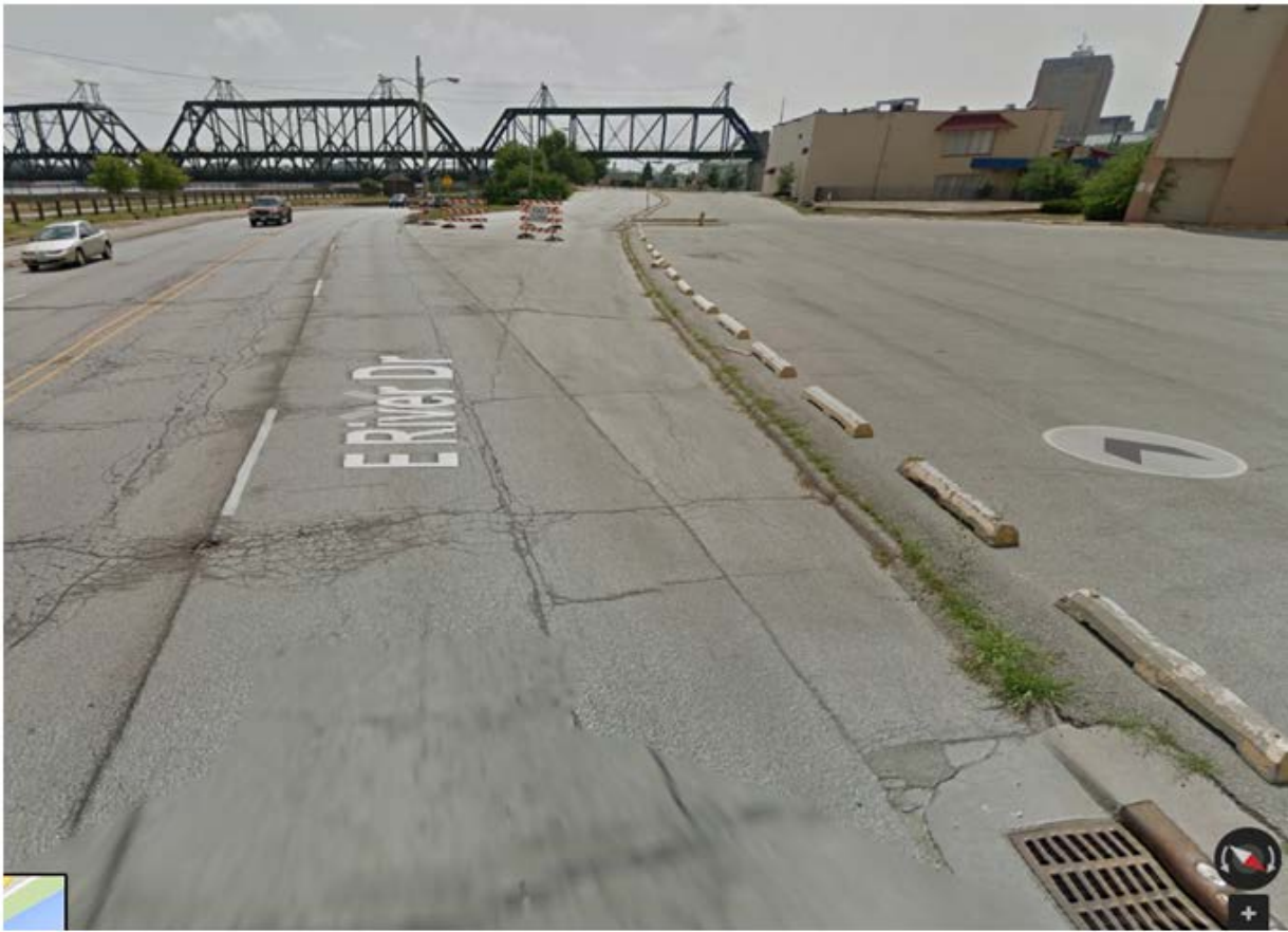
View to the west showing previous pavement 2 nd Street (barricaded)
