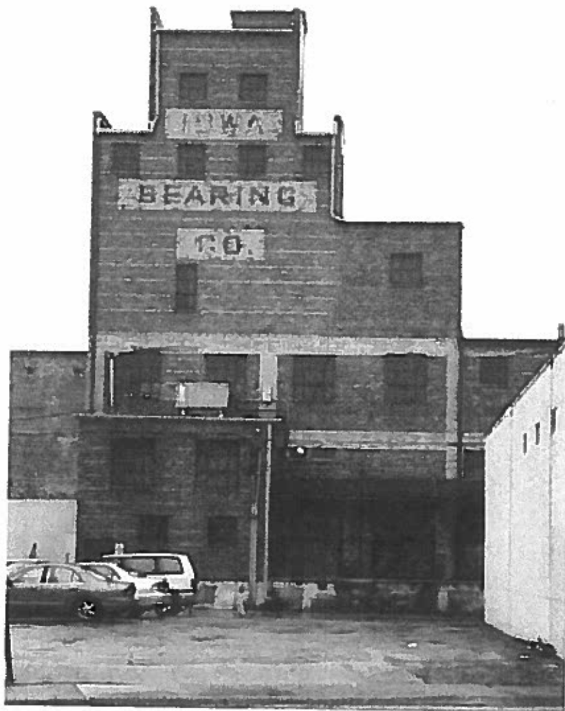
View of the rear (south) elevation.
