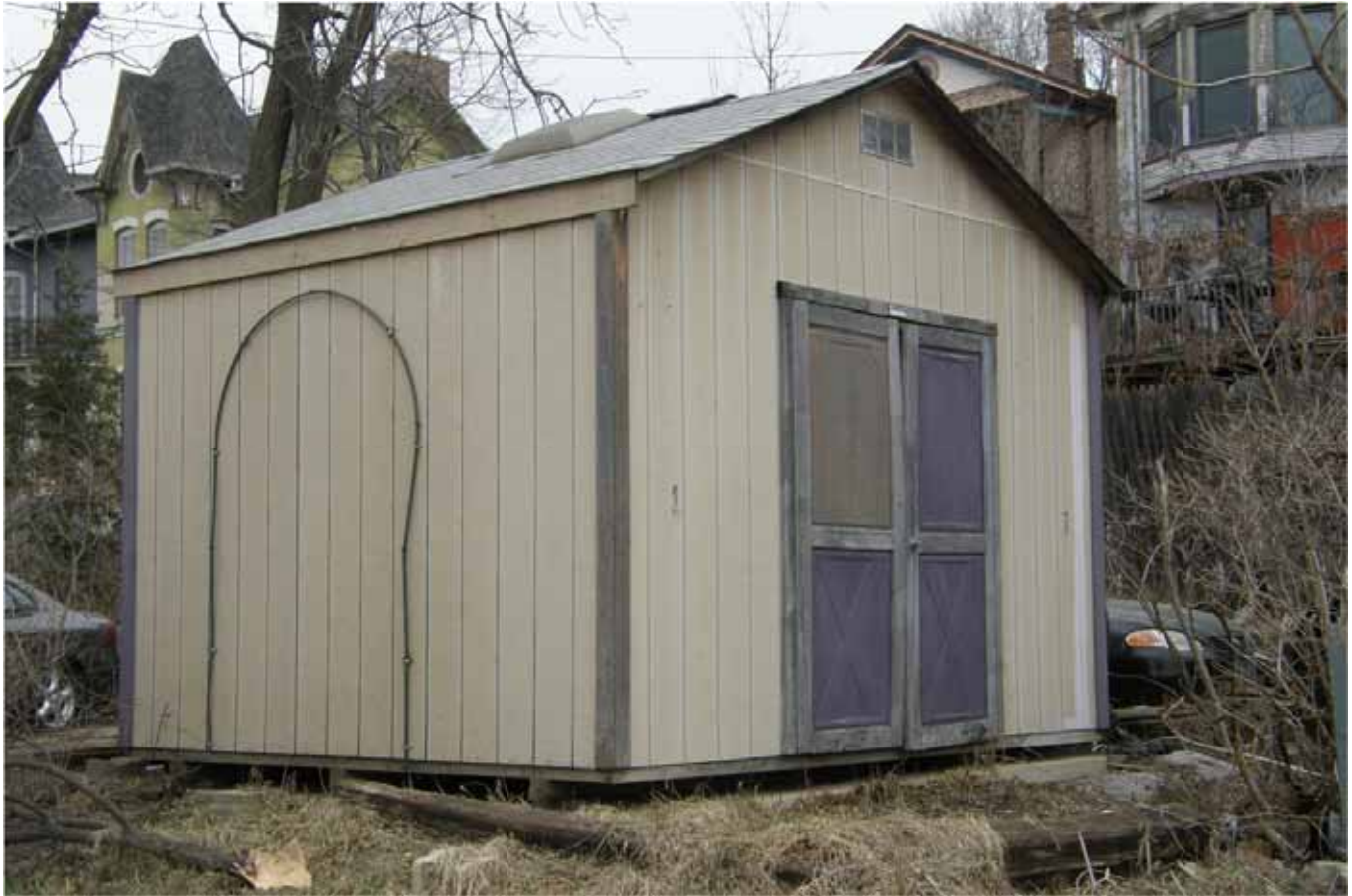
Photograph 82-00553-004 - Outbuilding, looking northwest (April 2015)
