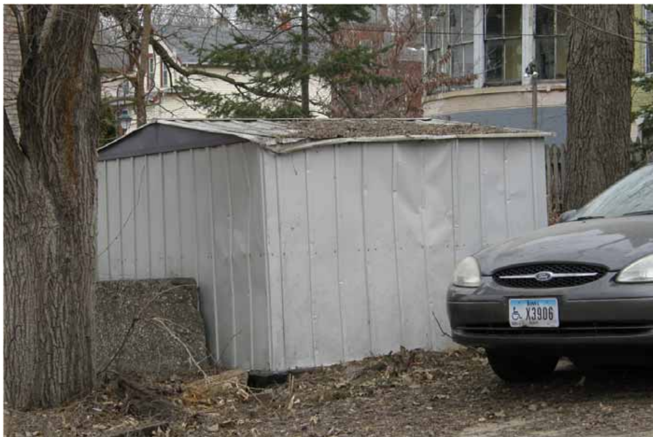
Photograph 82-00553-005 - Outbuilding, looking northwest (April 2015)
