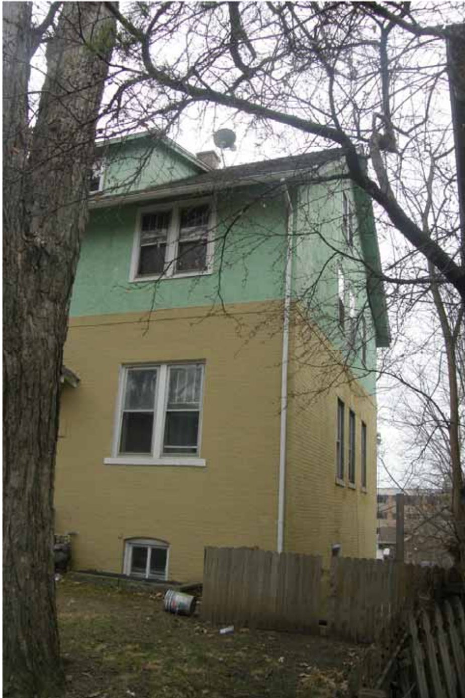
Photograph 82-00552-002 - House, looking southeast (April 2015)
