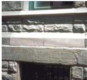
Replacement stones tooled to match original.
