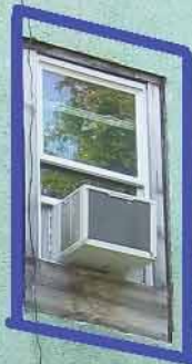
Windows have already Been Replaced, but will be replaced with custom Fit Double Hung Vinyl Windows.
