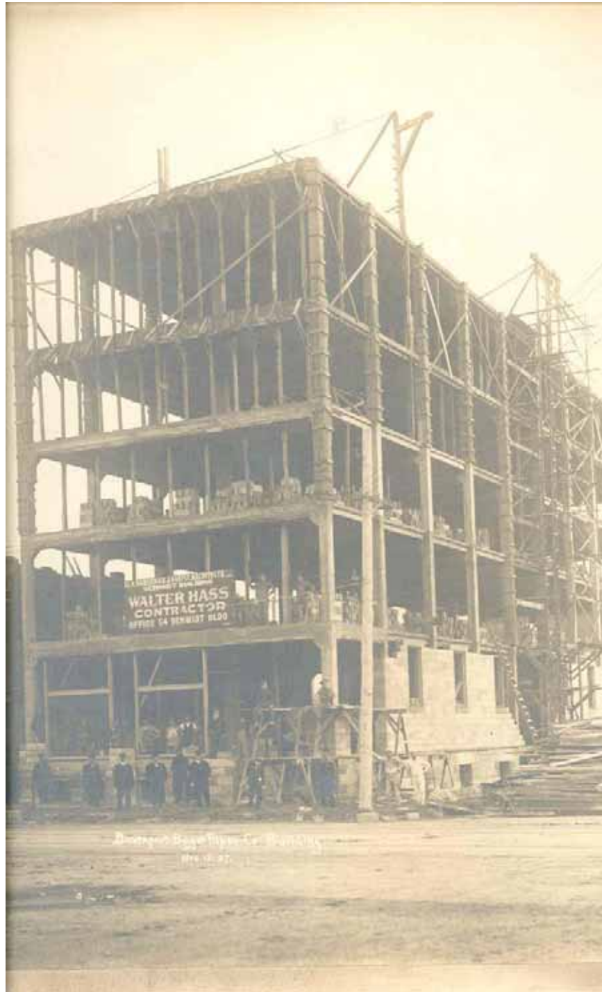
Wood-framed concrete column construction; site sign indicating contractor and architect, looking south. (Source: Valley Construction Co., April 2014)
