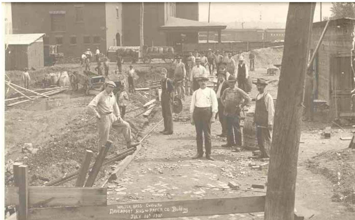
Construction beginning, July 10, 1907 (Source: Valley Construction Company, April 2014)
