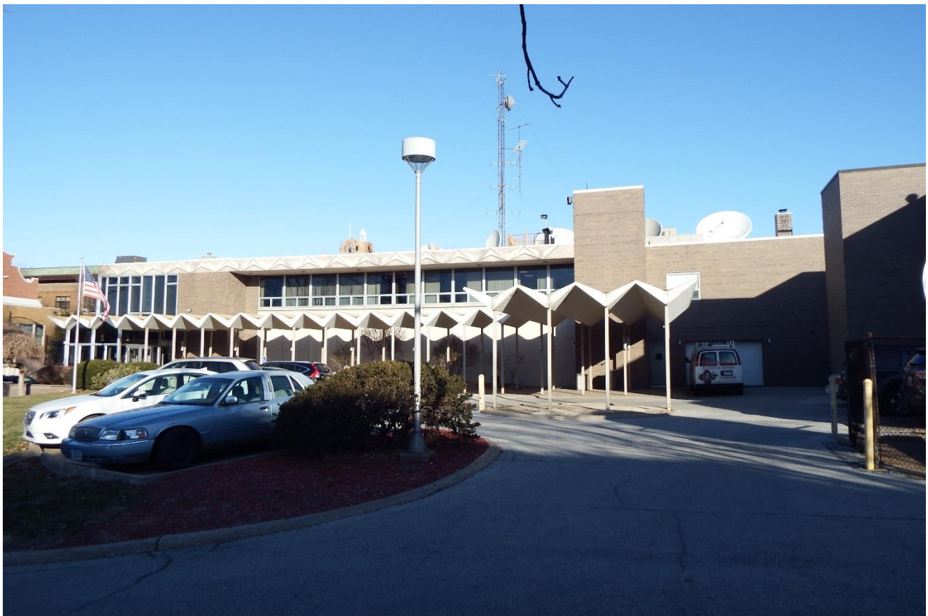
Photo 6: Exterior south façade, canopy, parking, looking northwest
