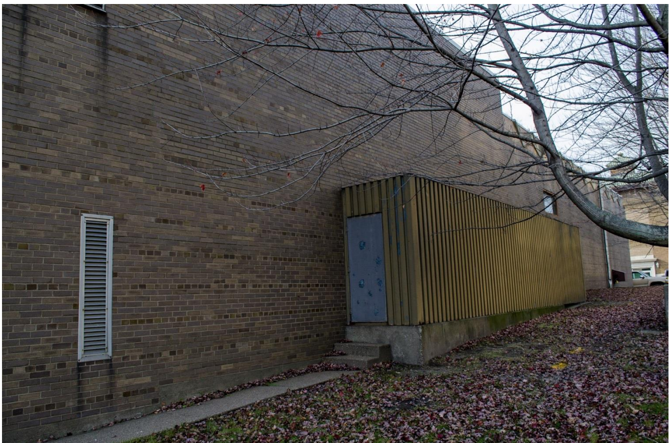
Photo 12: Exterior, north wall, looking southwest
