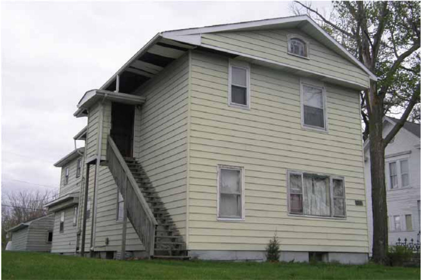
Photograph 82-06970-001 - House, looking northeast (April 2015)
