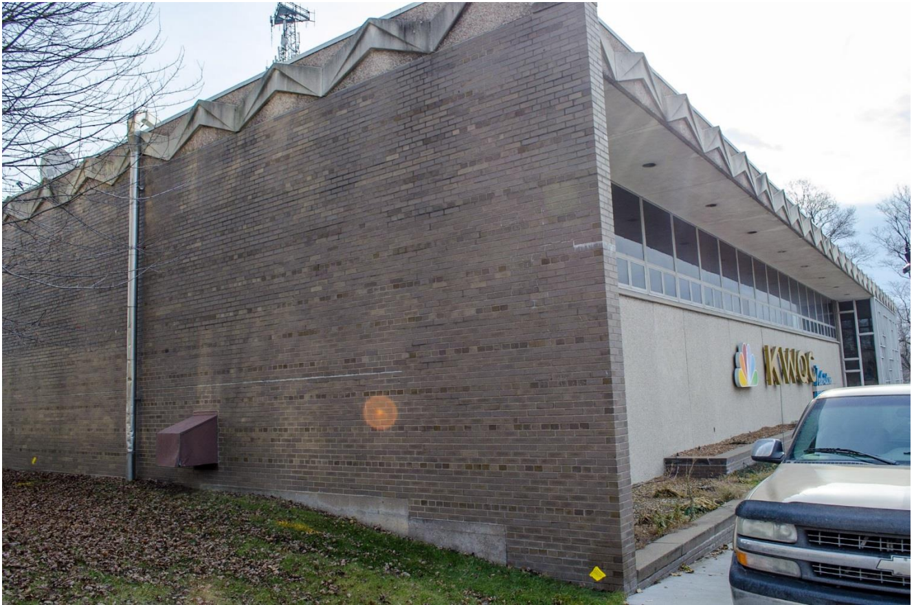
Photo 13: Exterior, north wall, west façade, looking southeast
