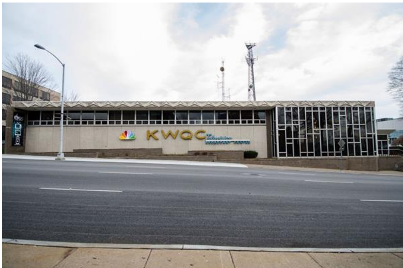
Photo 2: Exterior west façade detail, looking southeast
