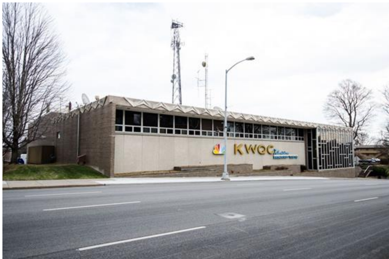
Photo 1: Exterior west façade, looking southeast
