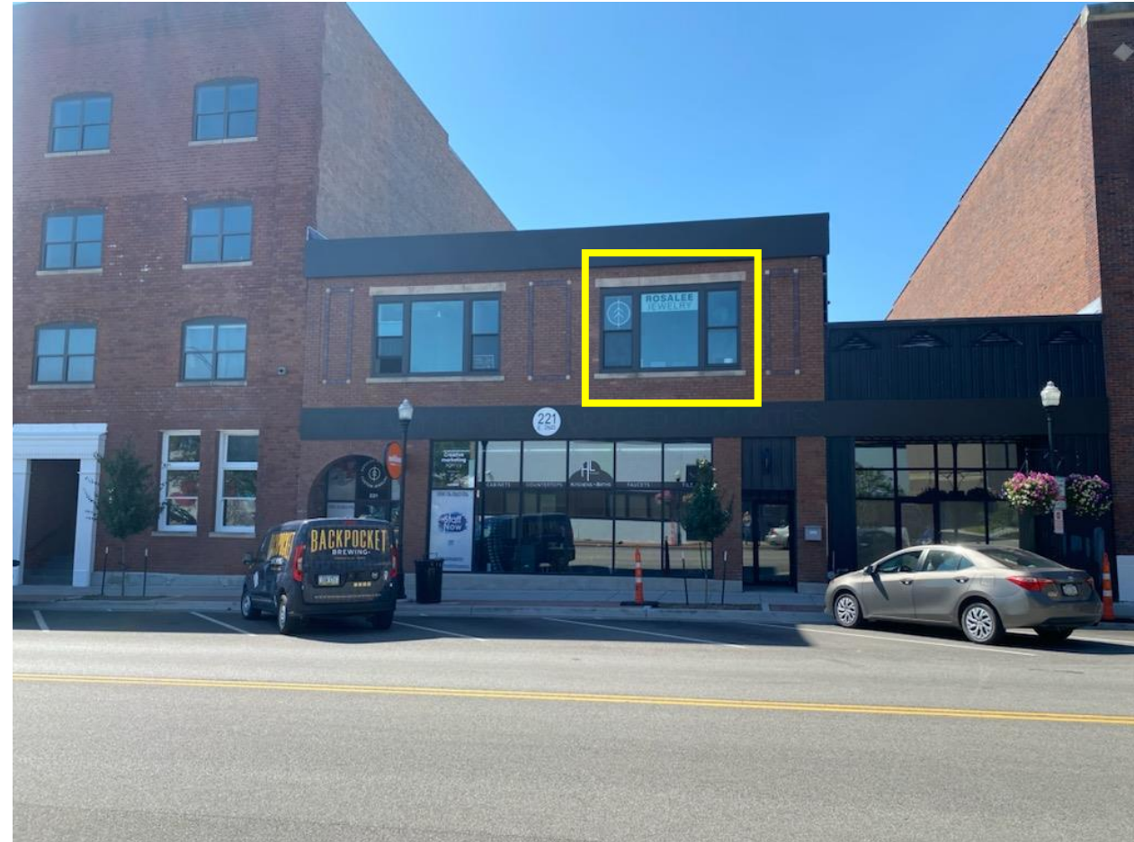
Existing Window Signage
