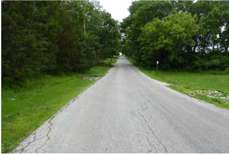
View of Vine Street, facing south
