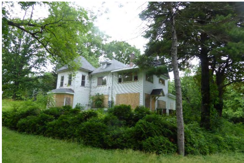
View of the duplex, facing northwest
