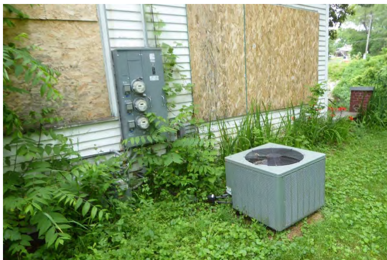
View of the air-conditioning condenser and electrical meters
