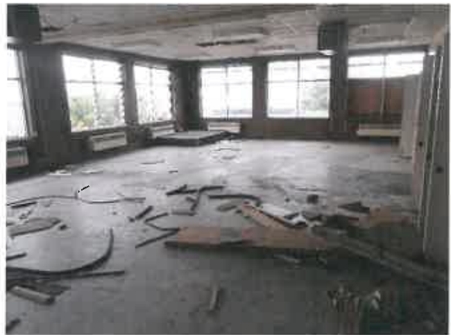
Upstairs Main room
