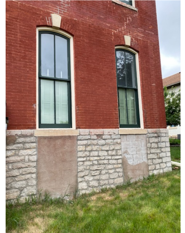
Install New Windows in Historic Openings
