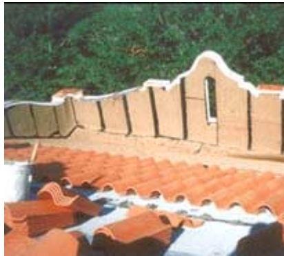
Replacement of damaged clay tile roof.
