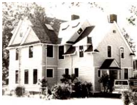
Non-obtrusive skylights on rear of residence.
