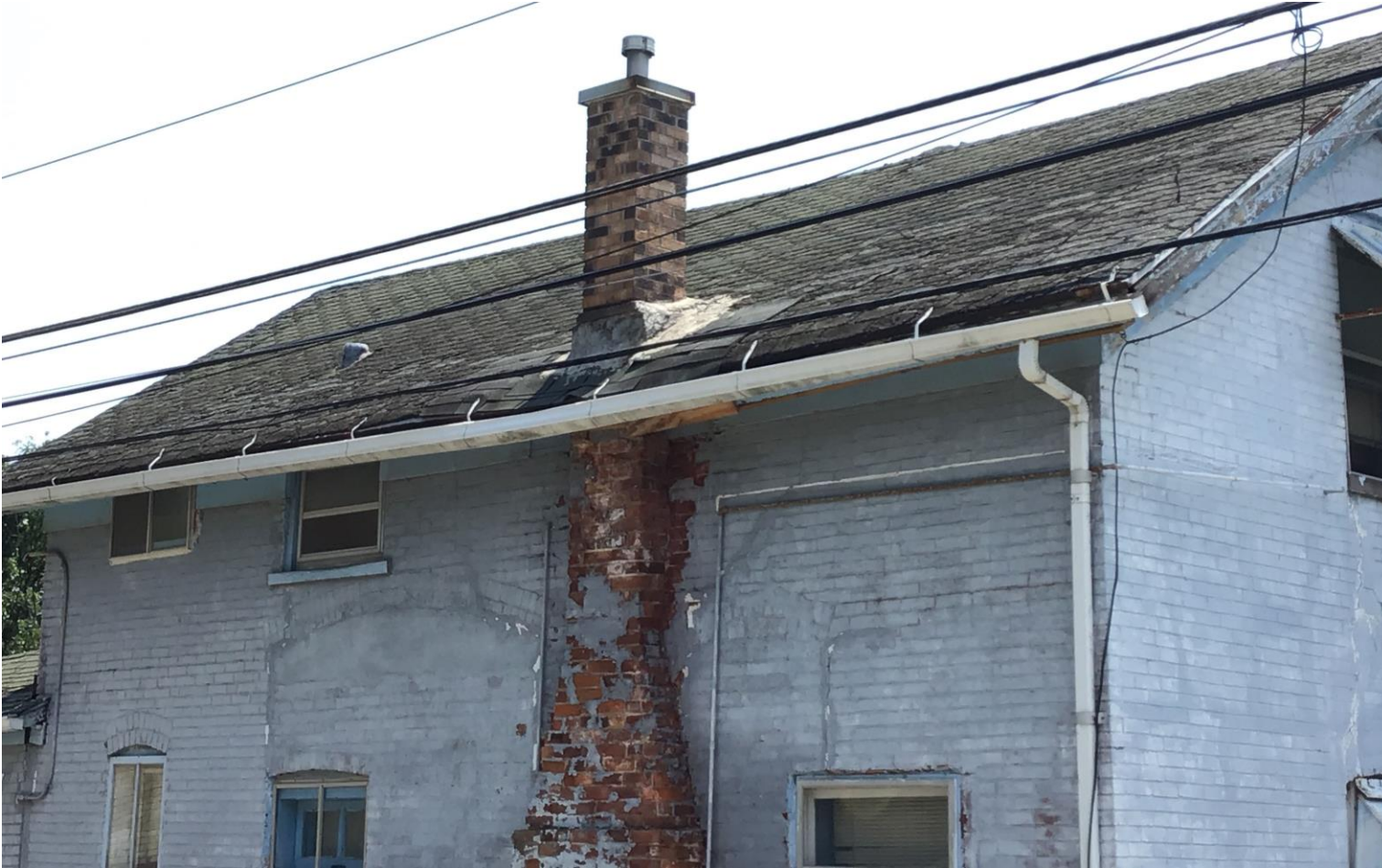
Gutters on Home (2021)
