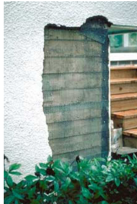
Preparation for stucco repair.
