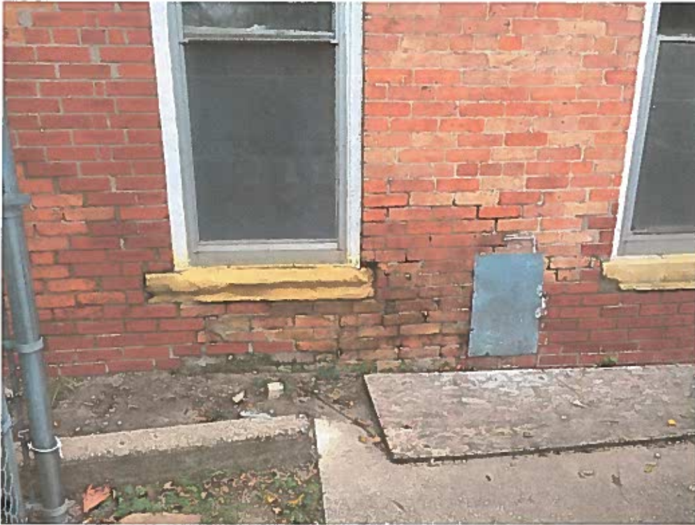
Deteriorated Brick
