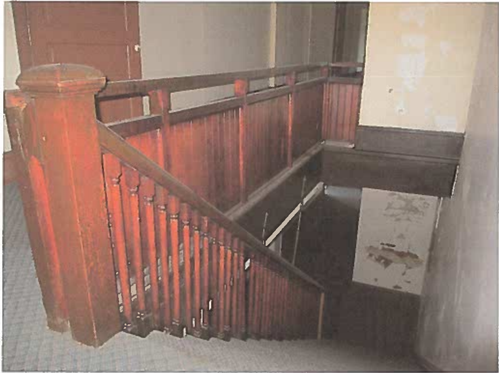
Third Floor – Open stair with 32" high guard railing
