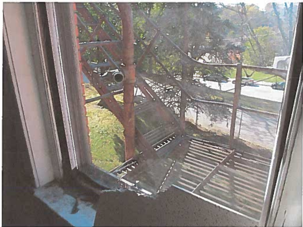
Second Floor – Window to exterior fire escape
