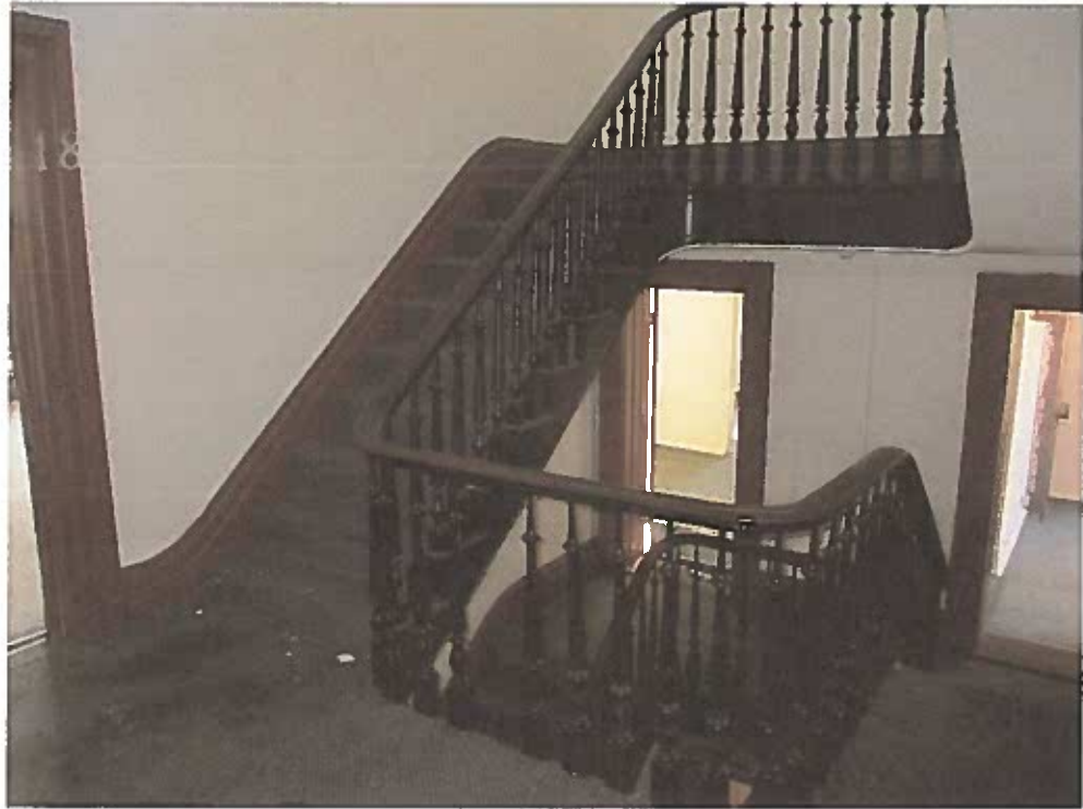
Second Floor – Open stair
