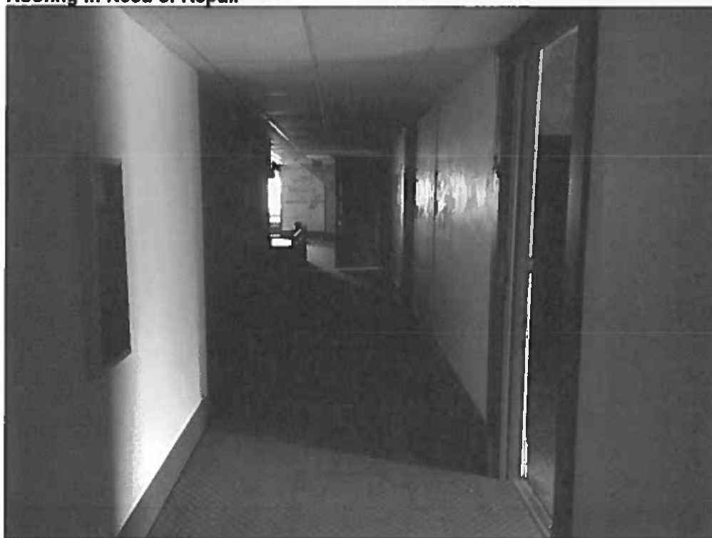
Sunken Corridor Area
