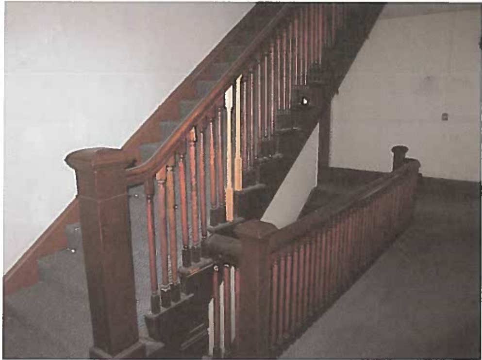
Second Floor – Open stair with 32" high guard railing
