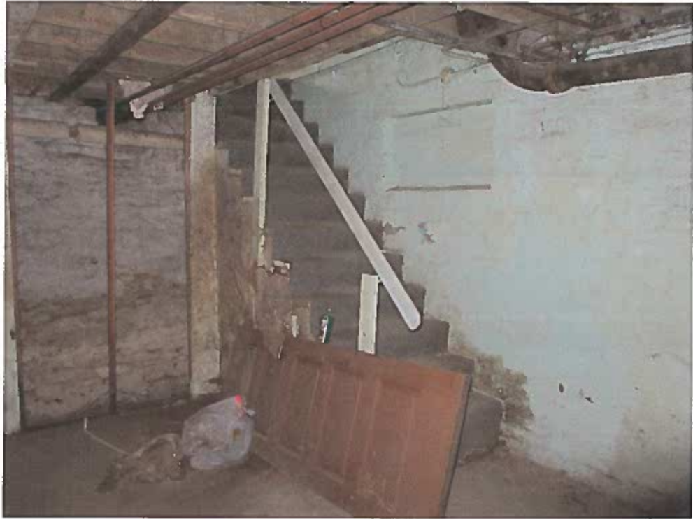
Basement – Stair to first floor
