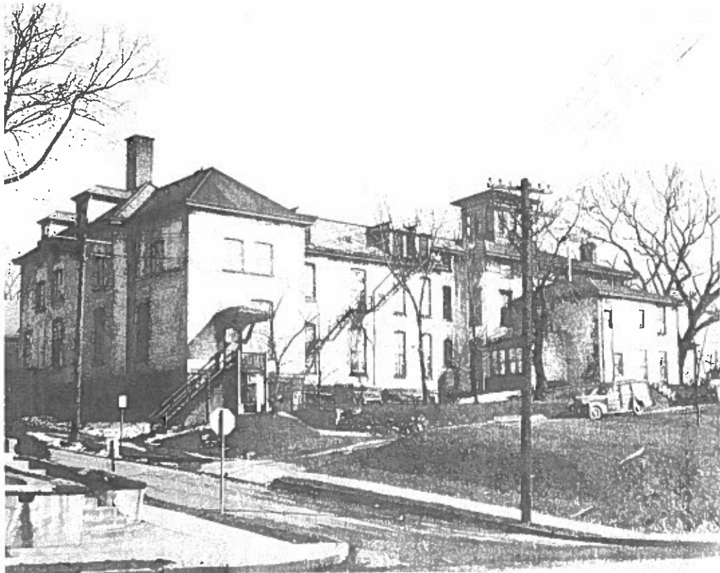
Today the original St. Luke's still stands at Eighth and Main — now an apartment building
