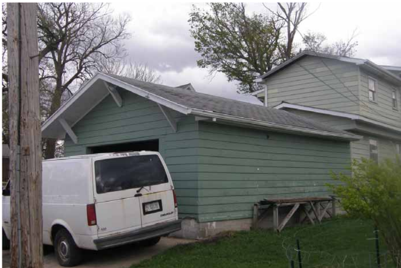
Photograph 82-06970-003 - Outbuilding, looking southeast (April 2015)
