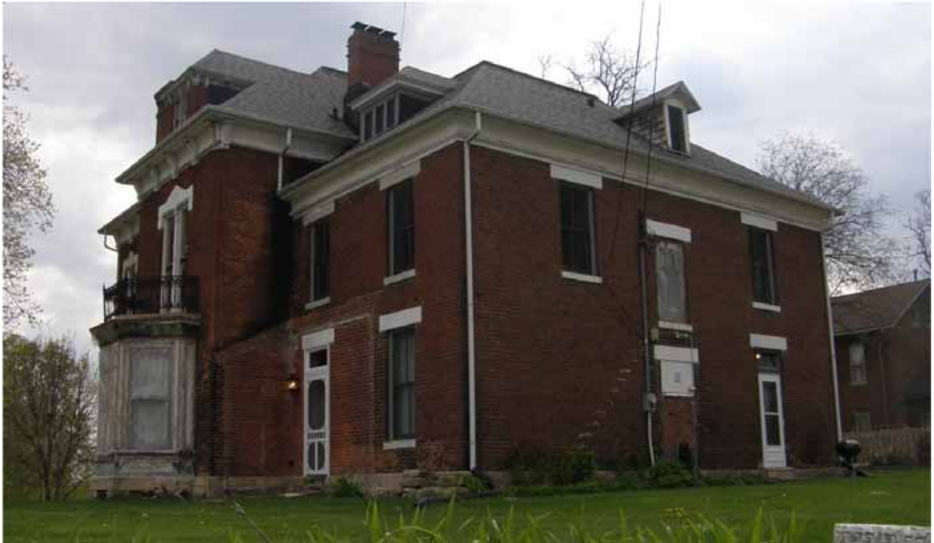
Photograph 82-00705-002 - House, looking southwest (May 2015)
