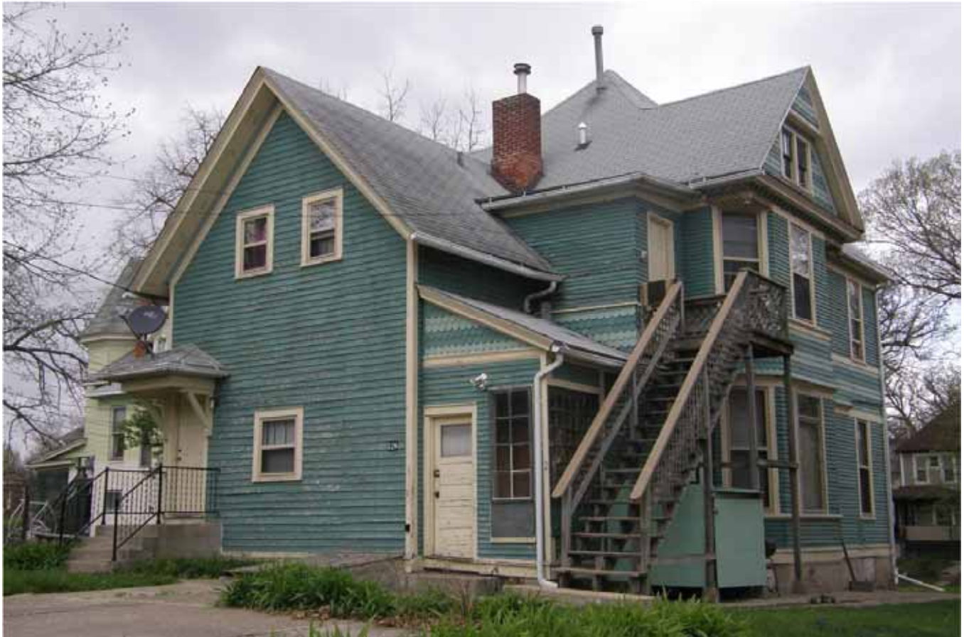
Photograph 82-00690-002 - House, looking northwest (May 2015)
