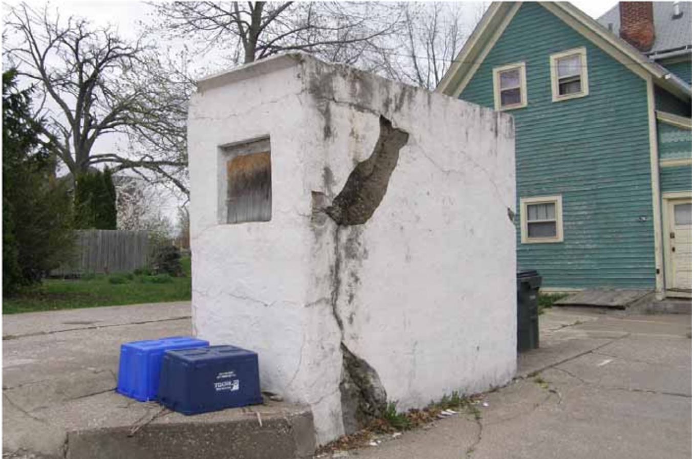
Photograph 82-00690-003 - Outbuilding, looking northwest (May 2015)
