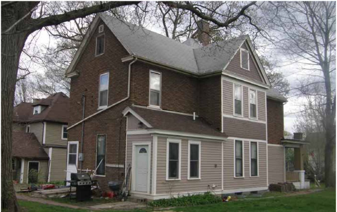
Photograph 82-00692-002 - House, looking southeast (April 2015)
