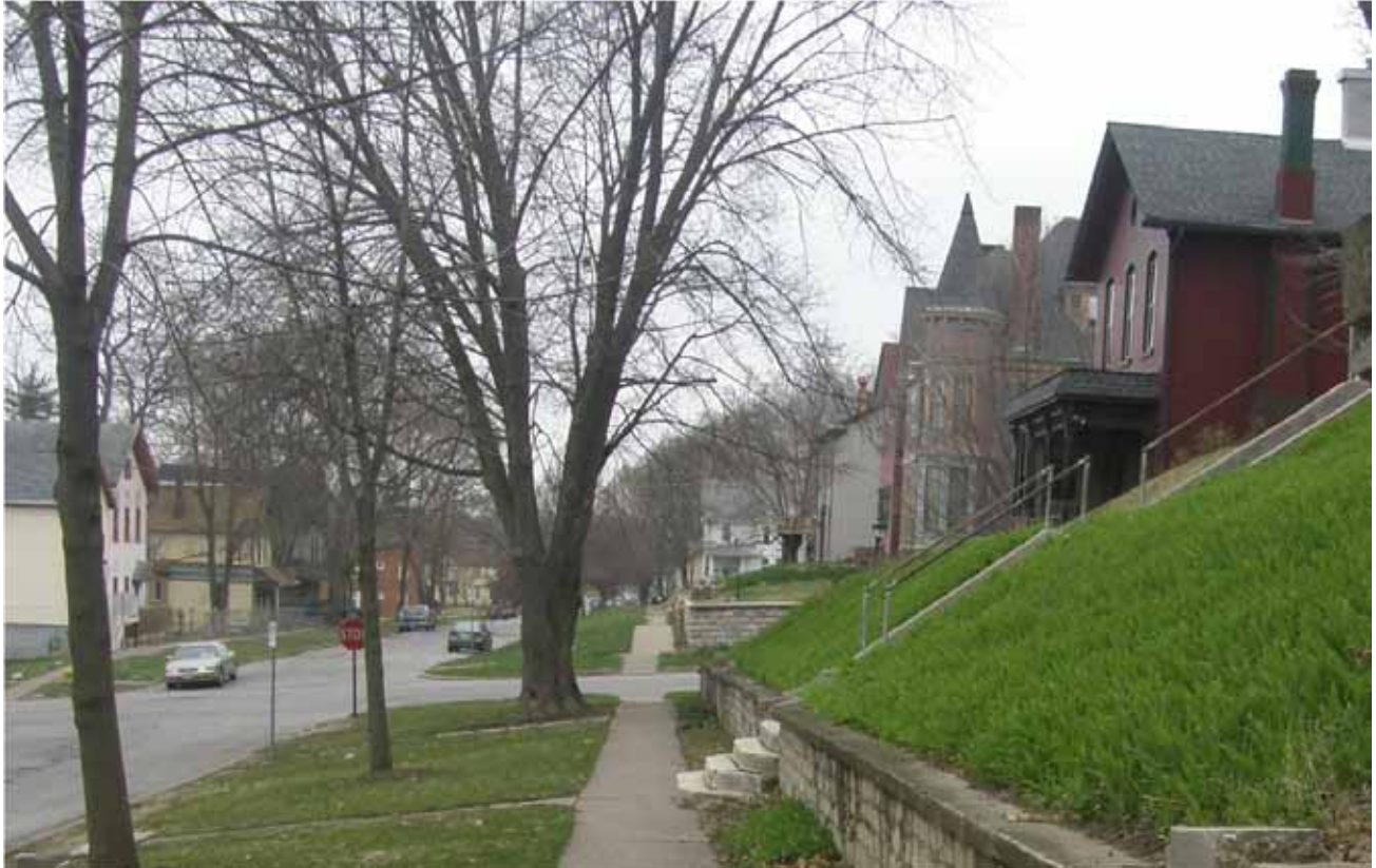
Photograph 82-00557-005 – Retaining wall, looking west (April 2015)
