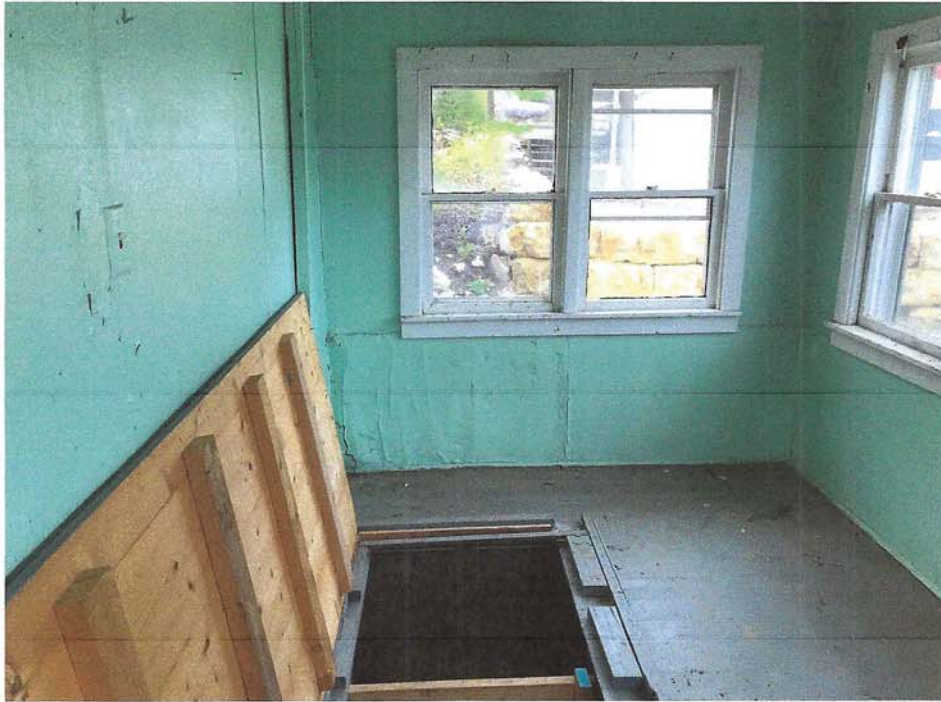
9. View of east addition with interior stairway.
