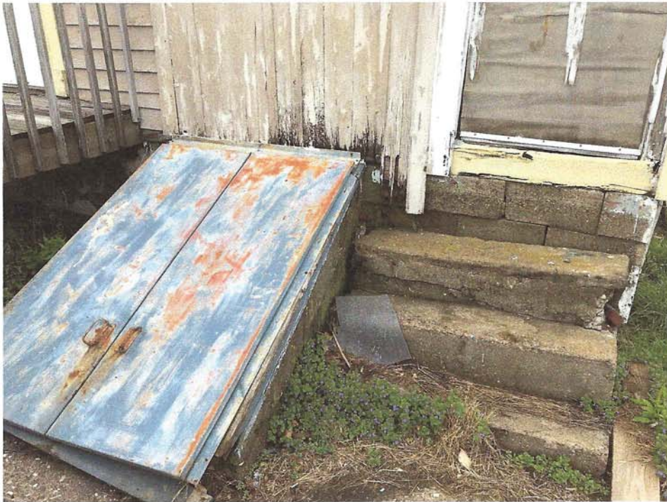
10. View of exterior stairs to basement.
