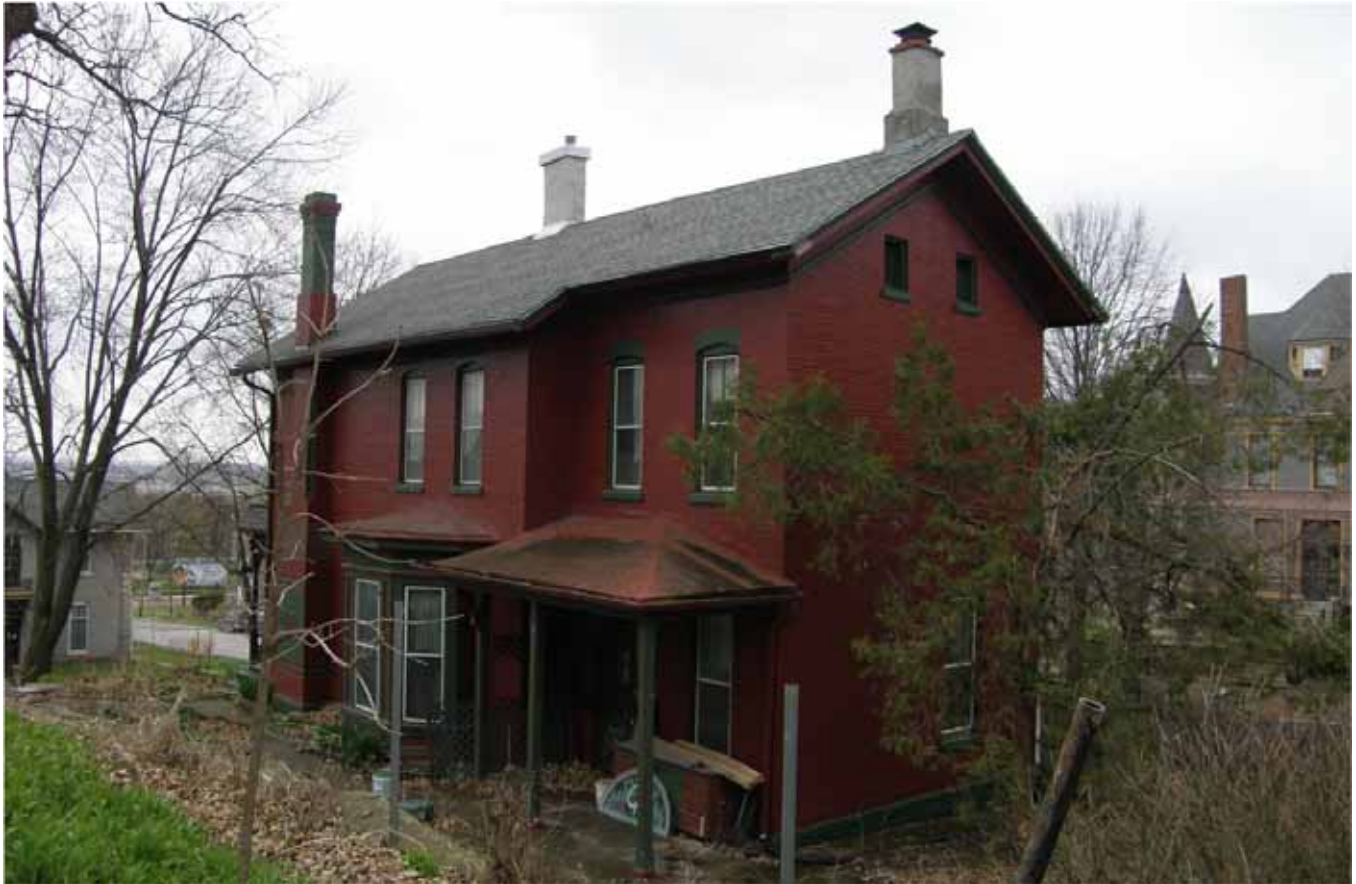
Photograph 82-00557-003 - House, looking southeast (April 2015)
