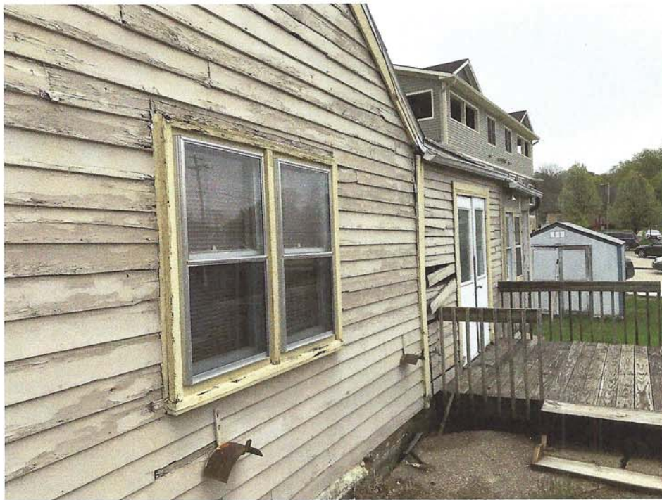
2. View of south side of house looking northeast.
