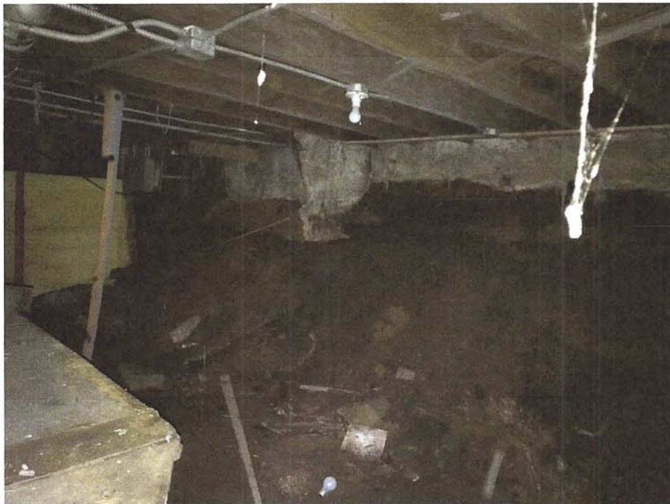
4. North stone foundation wall showing dirt and debris.
