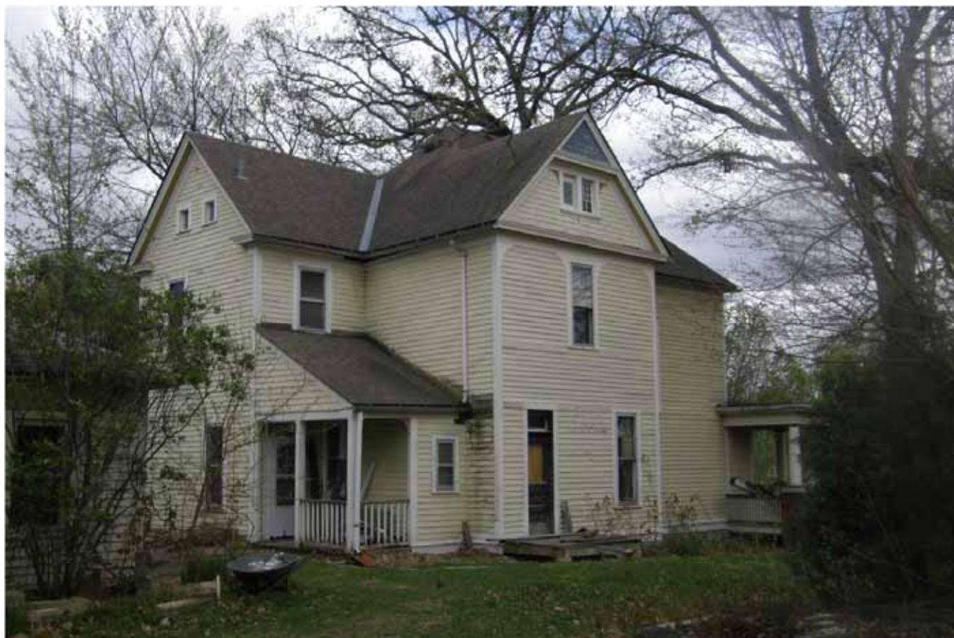
Photograph 82-00683-002 - House, looking southeast (April 2015)
