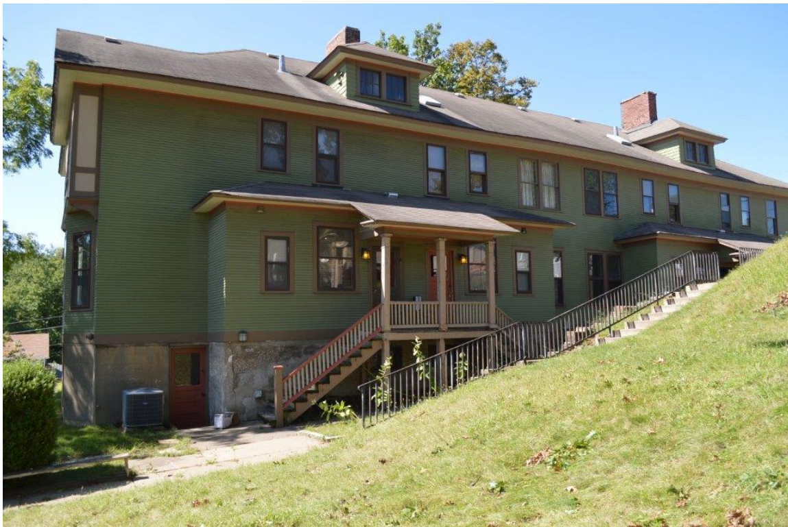
Looking NW, Louis P. Best Apartments, E elevation and roof condition.
