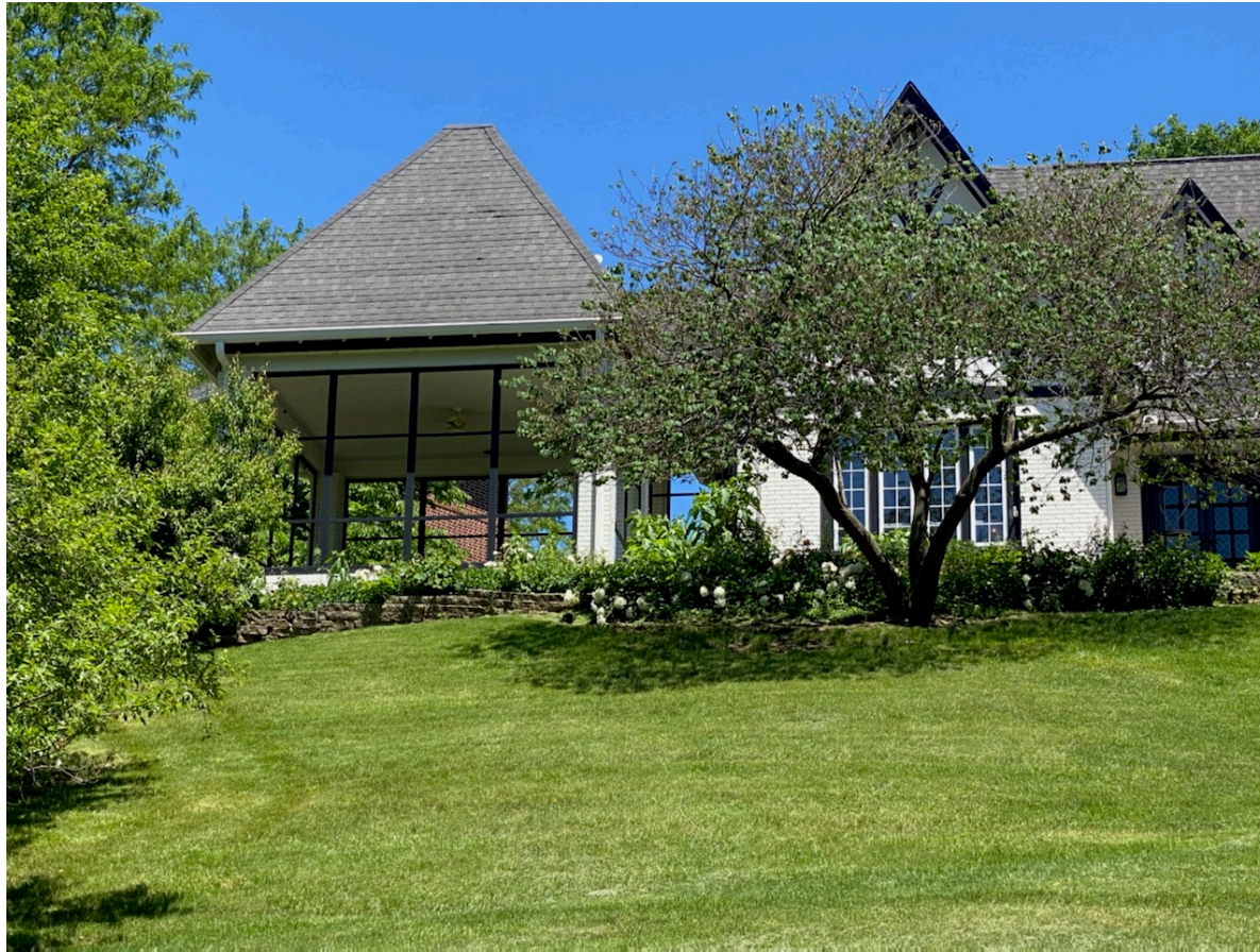
Screened Porch Proposed for Demolition
