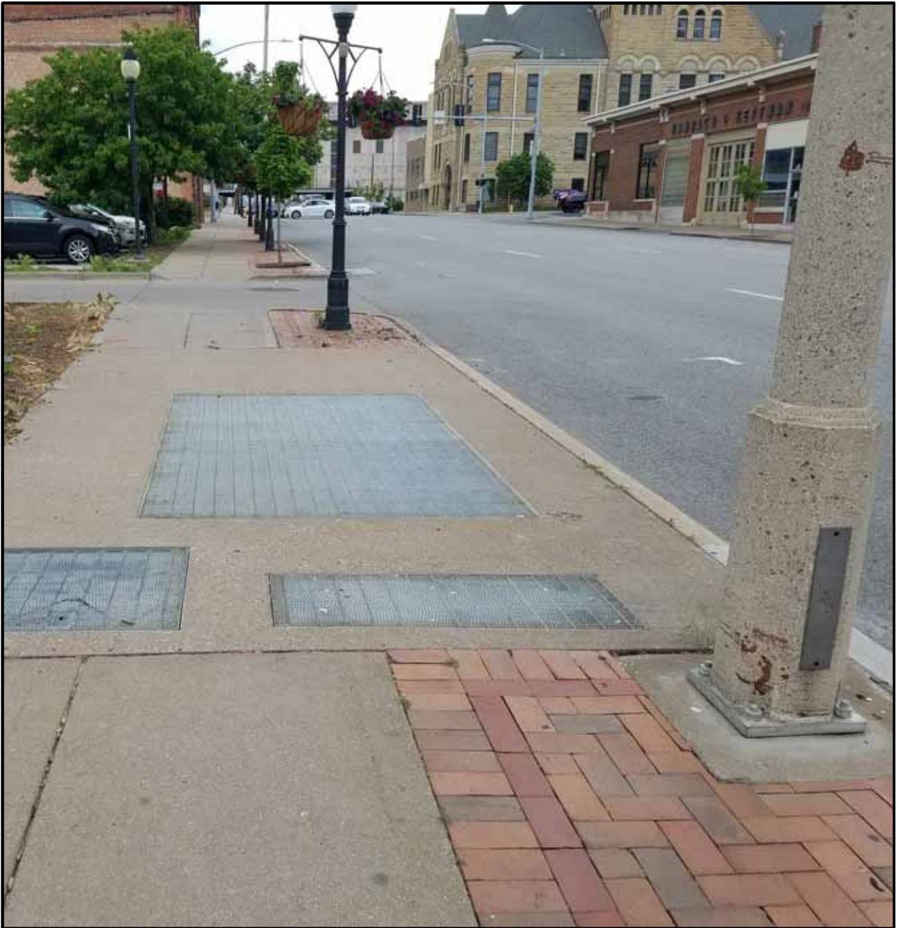
Figure 19. Utility vaults interrupting Streetscape on Harrison Street
