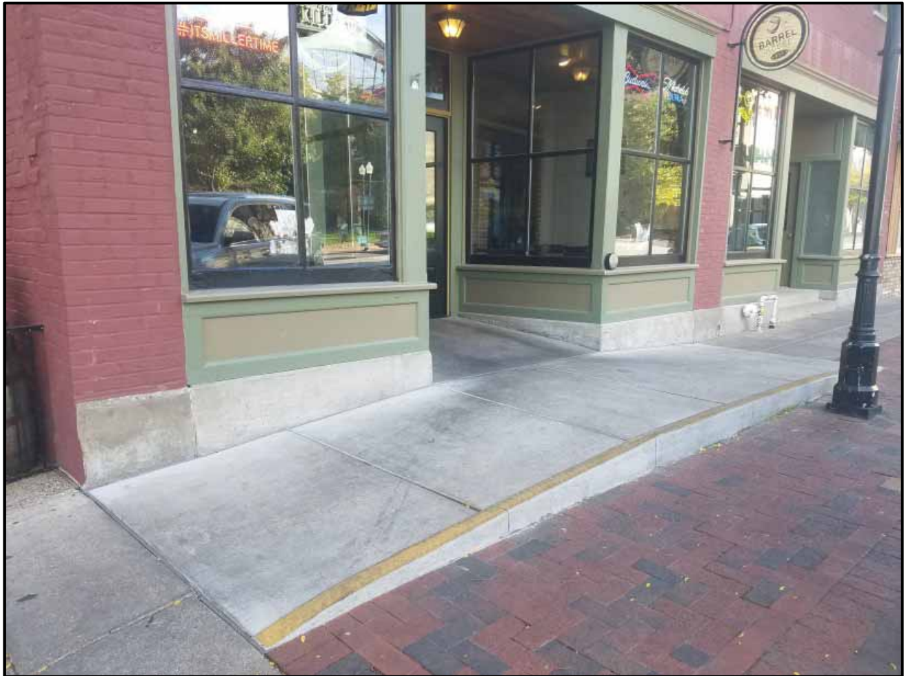
Figure 17. Accessible entrance to 211 East 2 nd Street
