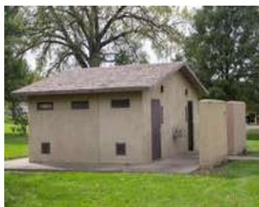
Marquette Park restroom
