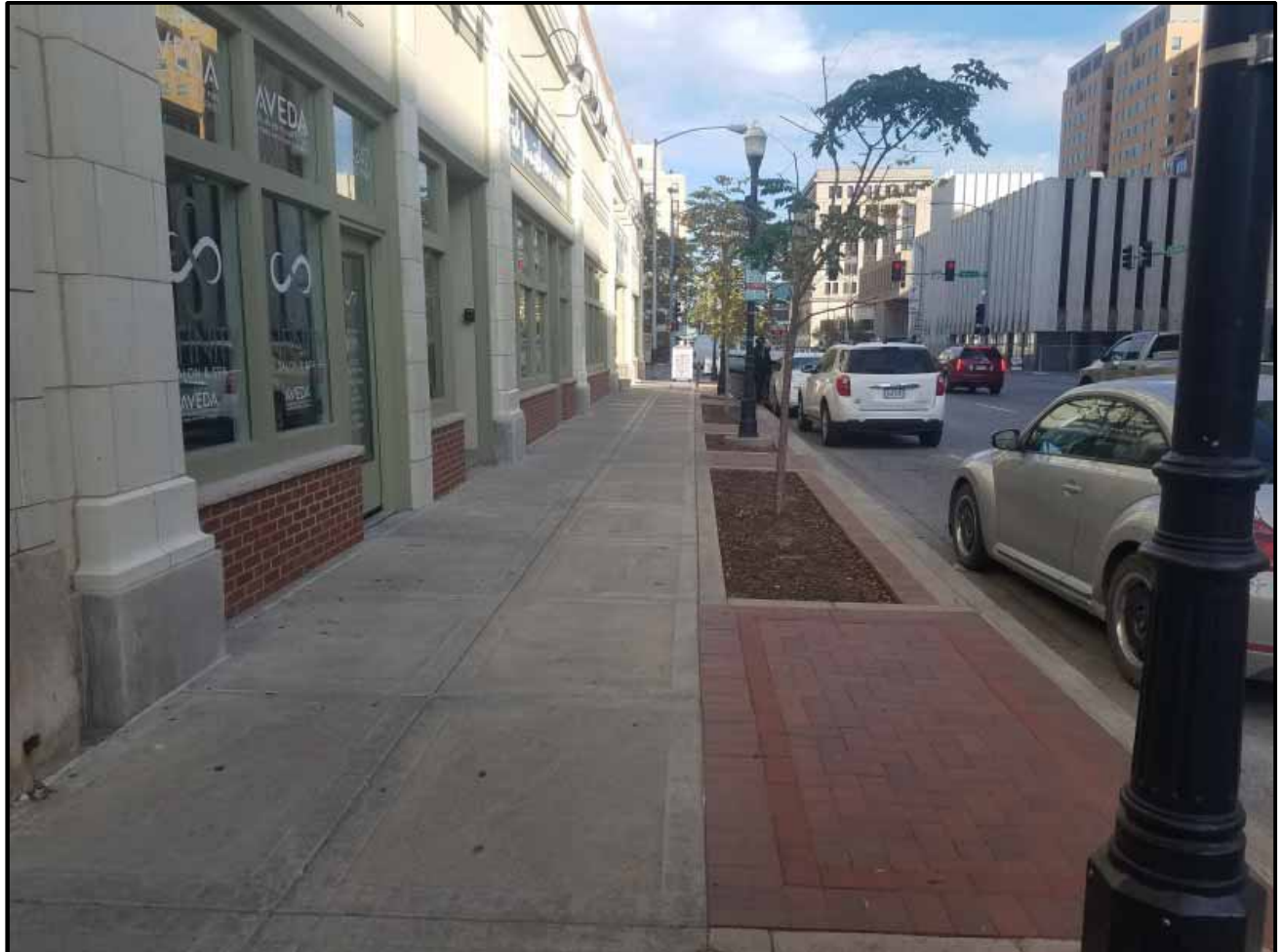
Figure 15. Sidewalk along West 3 rd Street
