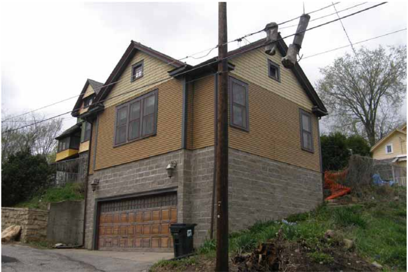
Photograph 82-01378-003 - Outbuilding, looking northwest (April 2015)
