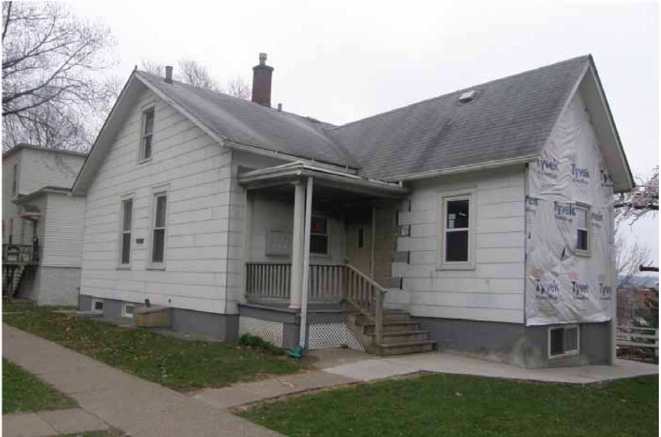
Photograph 82-00548-002 - House, looking southeast (April 2015)
