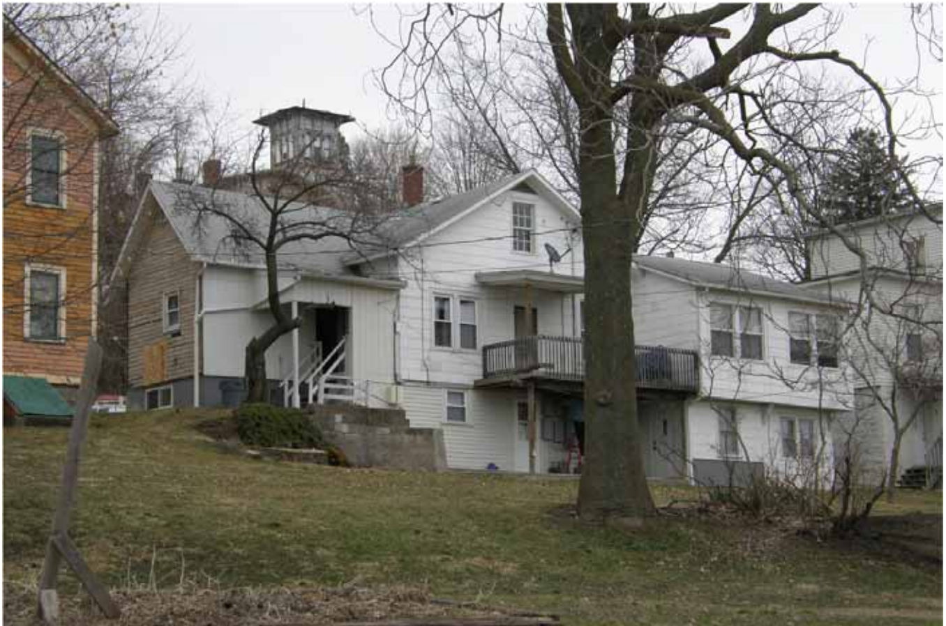
Photograph 82-00548-003 - House, looking northeast (April 2015)
