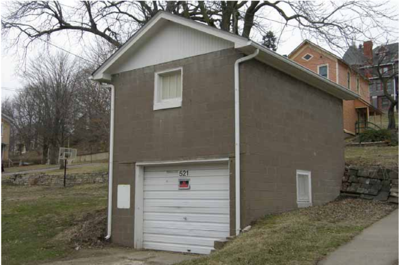
Photograph 82-00548-004 - Outbuilding, looking northwest (April 2015)
