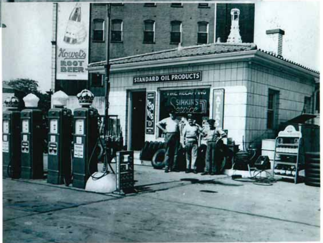
Former North elevation of Standard Hotel circa 1940
