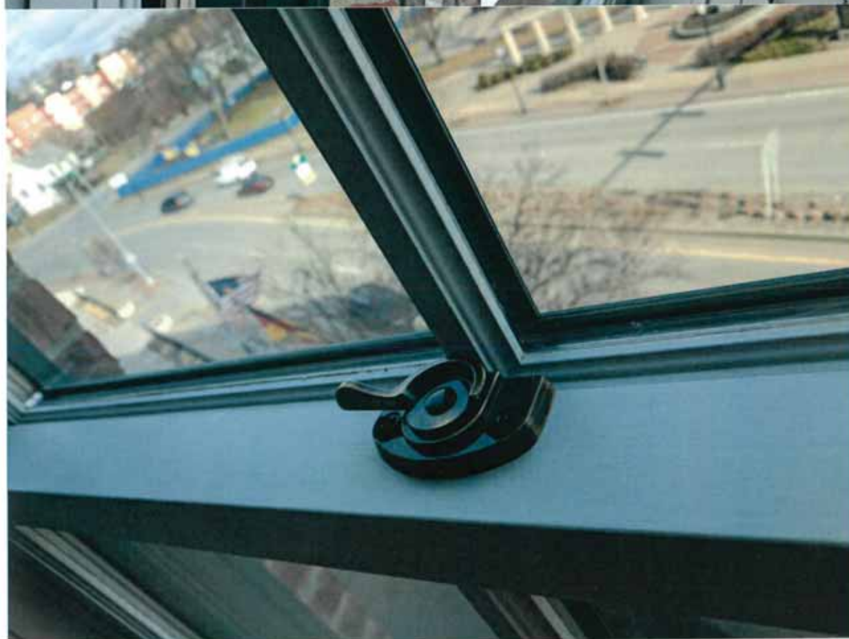
2017 new Marvin windows on 4th floor— will use same product for east elevation 2nd and 3rd floors
