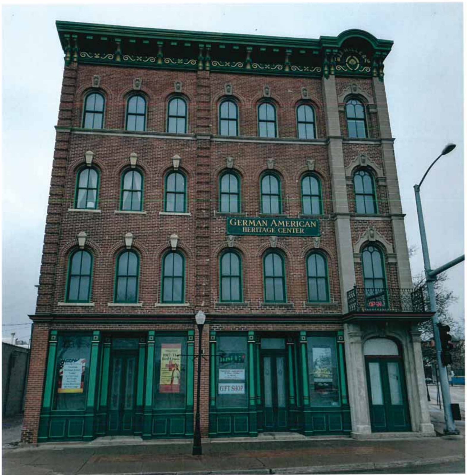
South façade 2017 – no work taking place here currently– 4th floor windows have been replaced.
