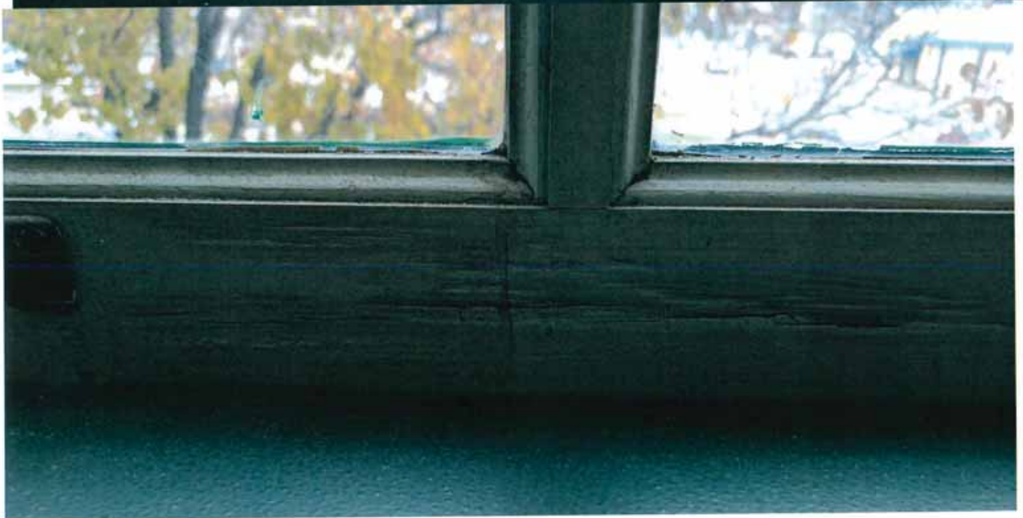
2016 eastern elevation— 2nd floor
