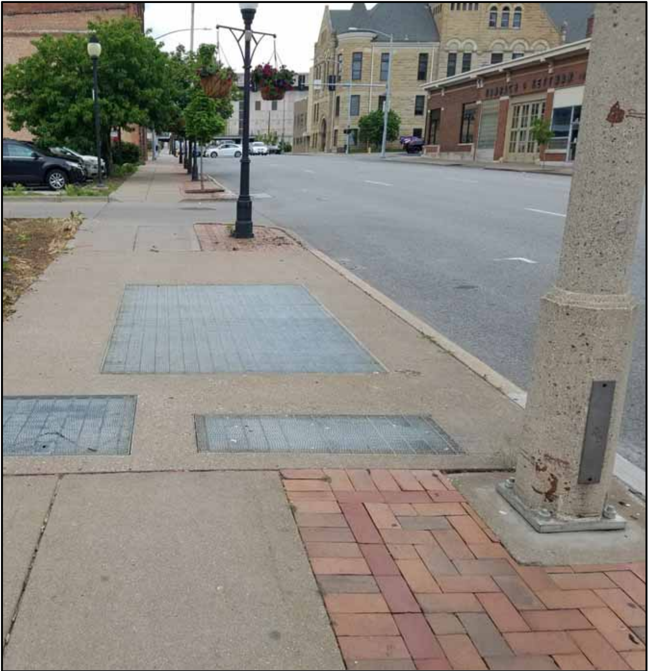
Figure 20. Utility vaults interrupting Streetscape on Harrison Street
