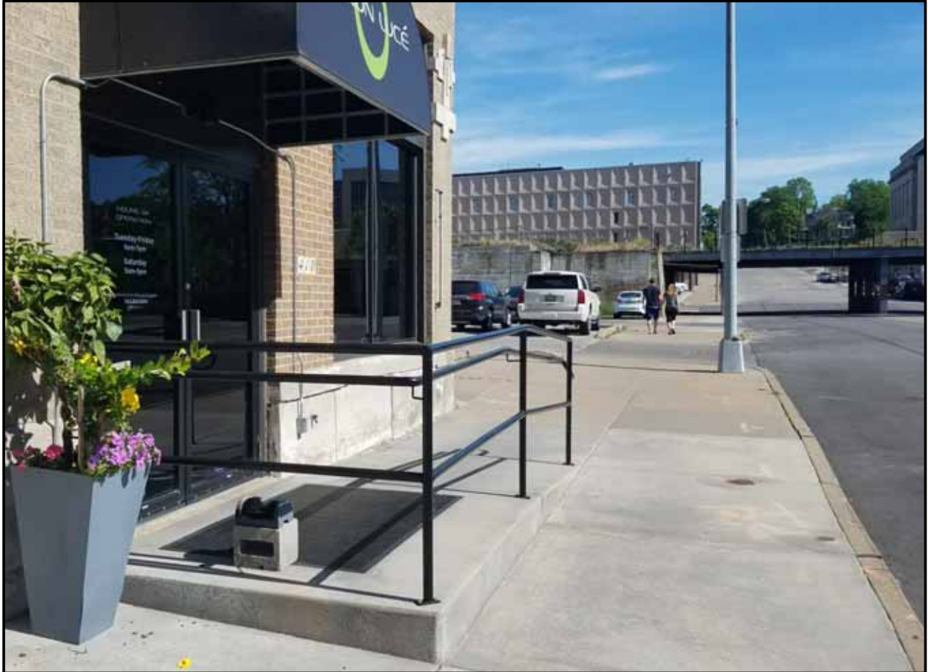
Figure 17. Accessible entrance to 402 East 4 th Street
