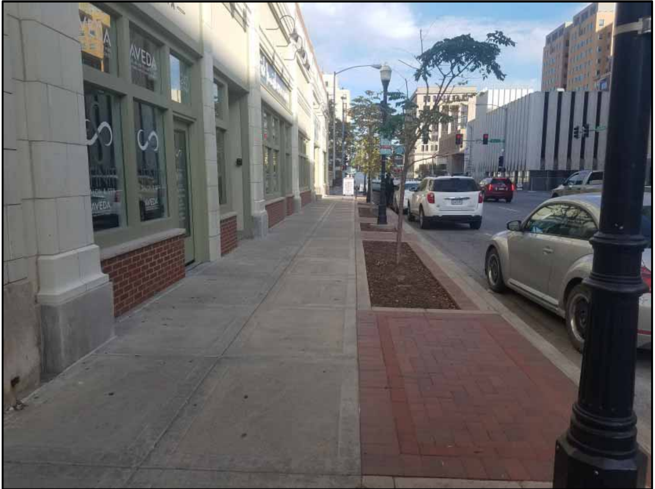
Figure 16. Sidewalk along West 3 rd Street
