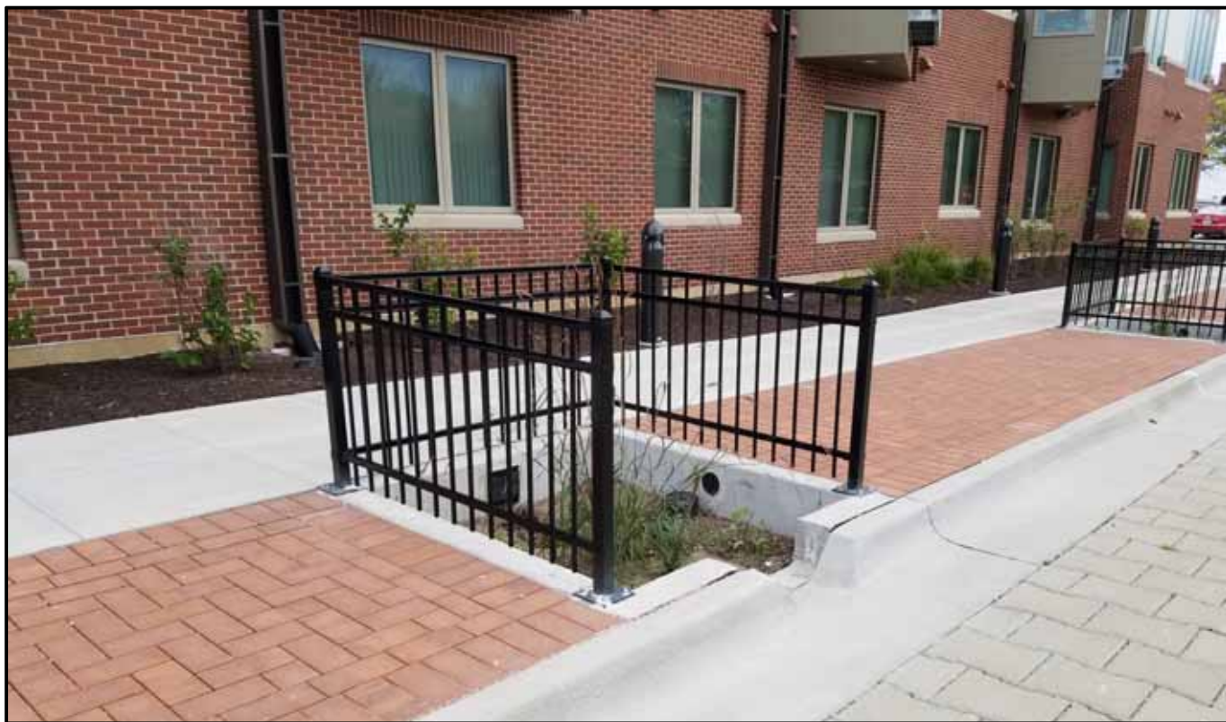
Figure 8. Tree well with Stormwater Management Feature
