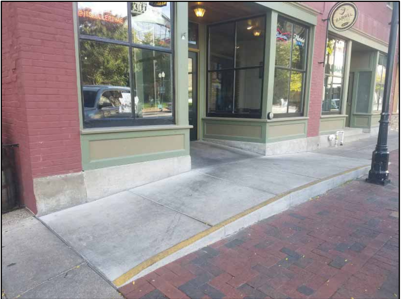
Figure 18. Accessible entrance to 211 East 2 nd Street
