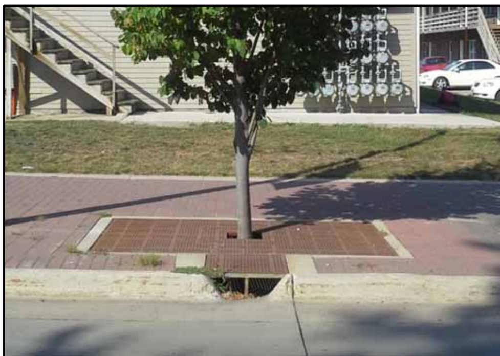
Figure 9. Tree well with Stormwater Inlet and Tree Grate
