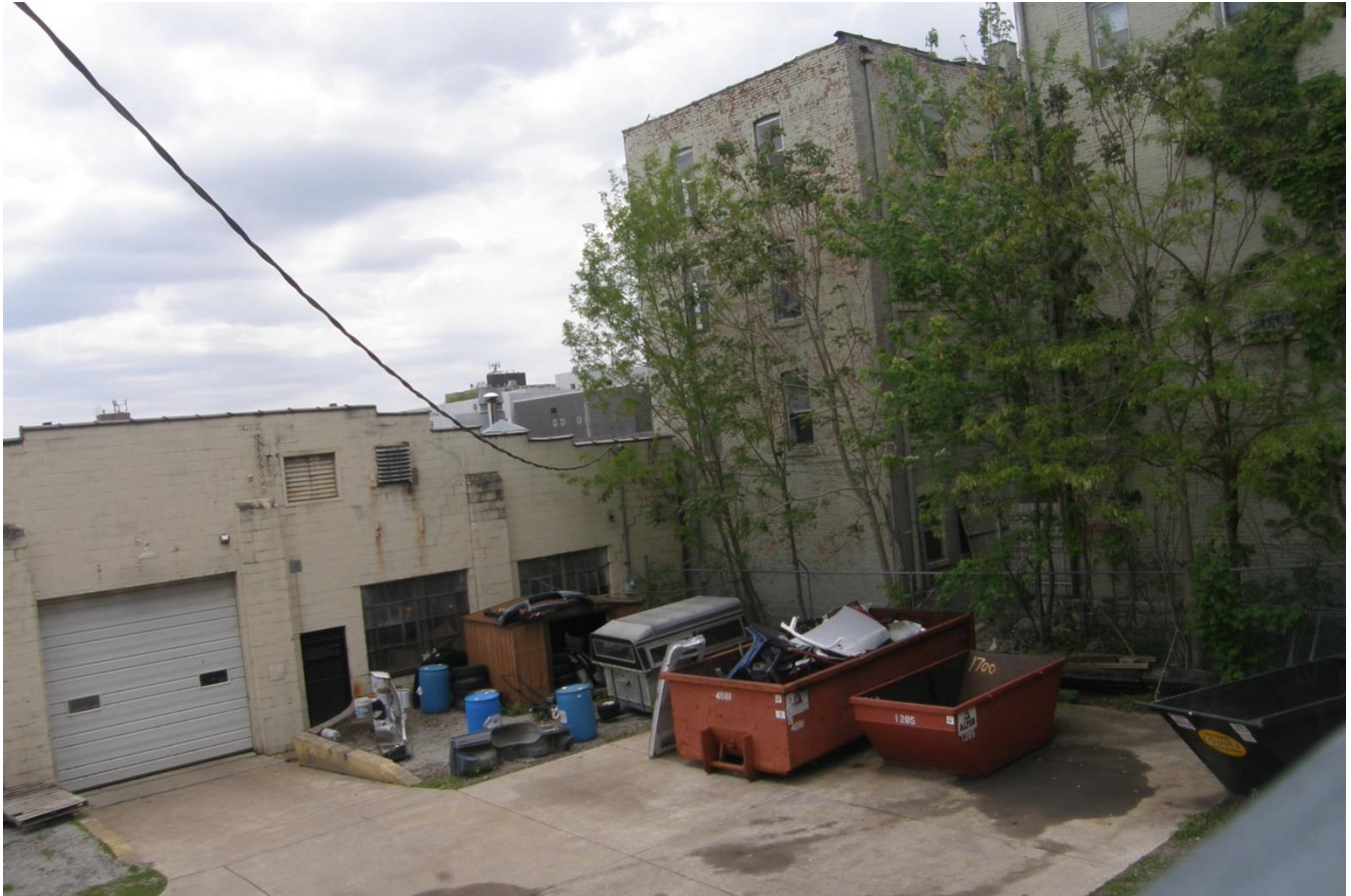
Photograph 82-02488-003 - Flats, looking southwest (May 2015)
