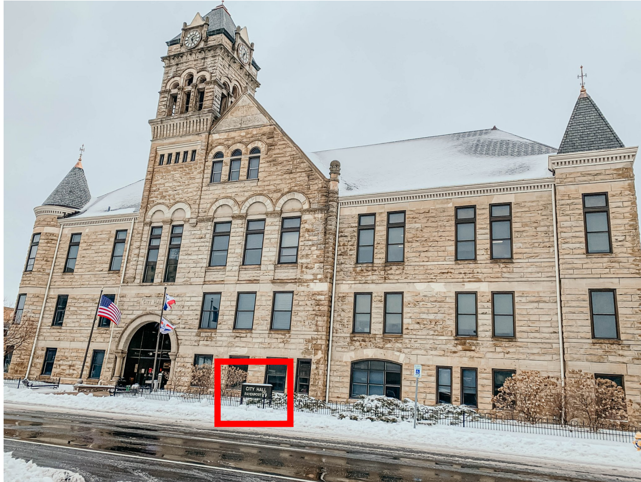
Existing City Hall Monument Sign to be Removed
