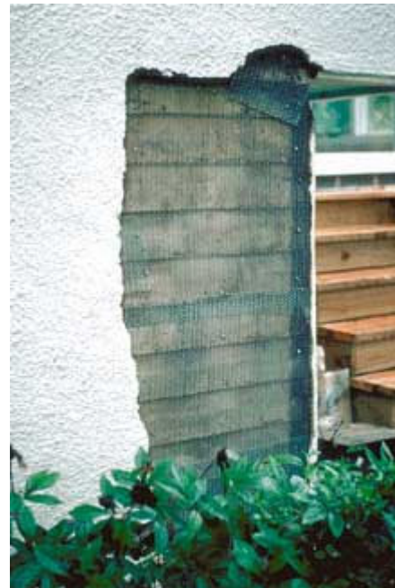
Preparation for stucco repair.
