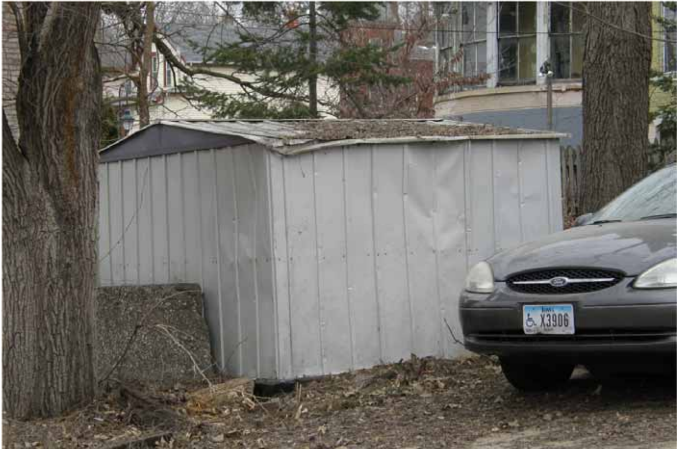
Photograph 82-00553-005 - Outbuilding, looking northwest (April 2015)
