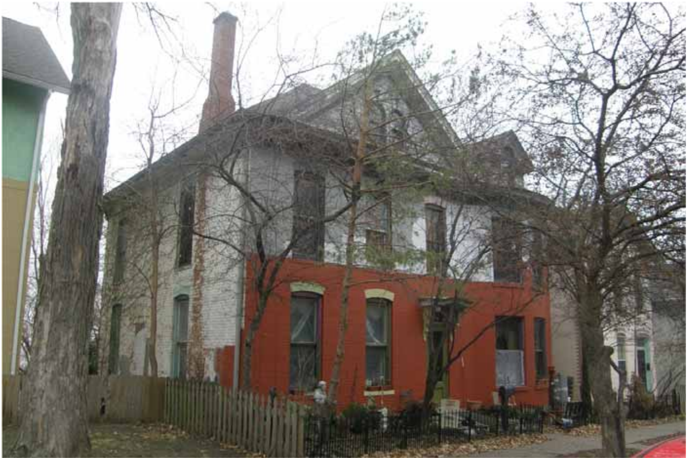
Photograph 82-00553-001 - House, looking southwest (April 2015)
