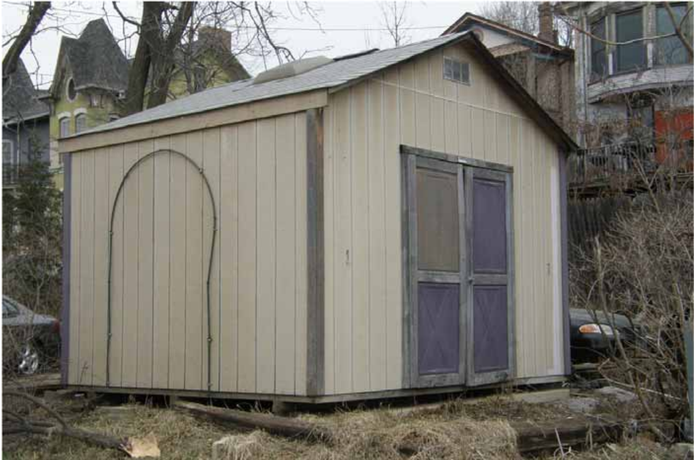
Photograph 82-00553-004 - Outbuilding, looking northwest (April 2015)
