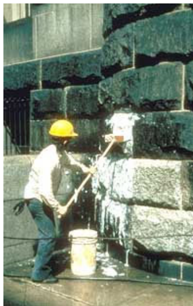
Chemical cleaning to remove dirt from granite.
