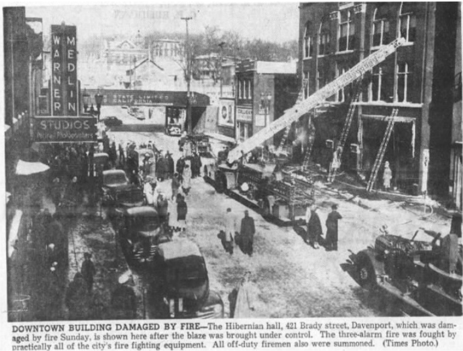
Figure: In the 1950s, fire damaged the old Hibernia Hall building in the 400 block of Brady Street. Note the elevated train viaduct over Brady Street in the background. (The Daily Times, December 24, 1951: 11)
