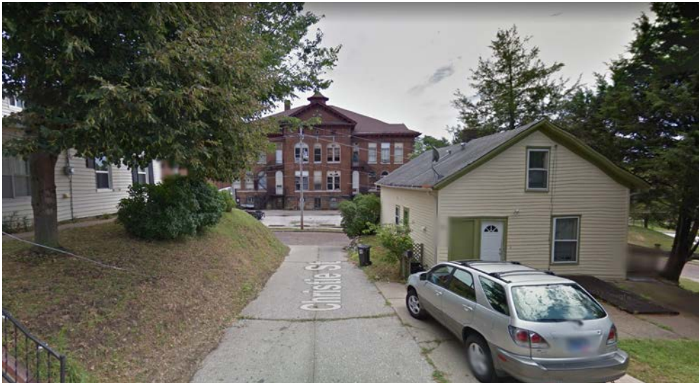
View From Alley - Facing East
