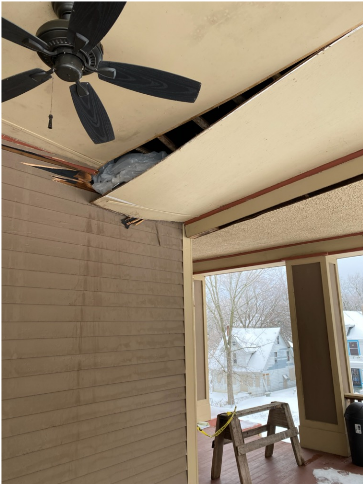
Stucco Ceiling to be Repaired and Painted to Match Existing Color & Material
