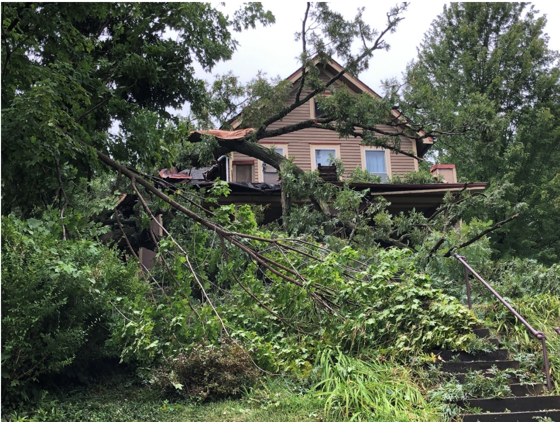
Tree Damage from Derecho
