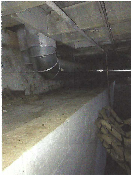
North block wall constructed in front of existing stone foundation.
