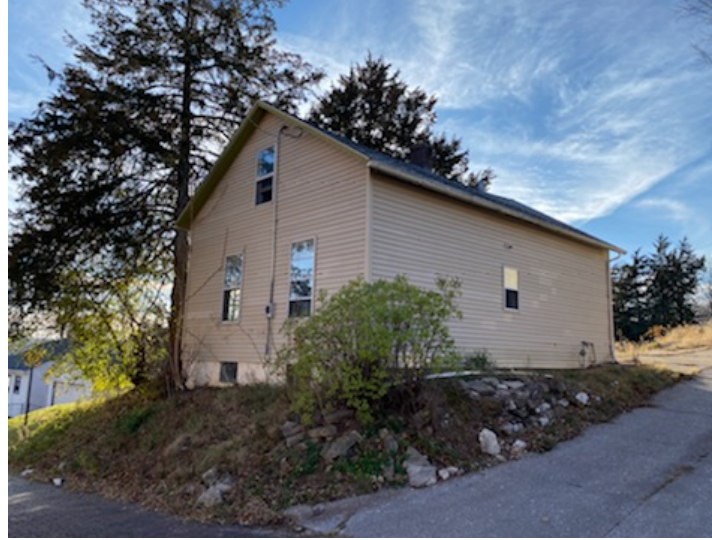
East Elevation-View From Christie Street
