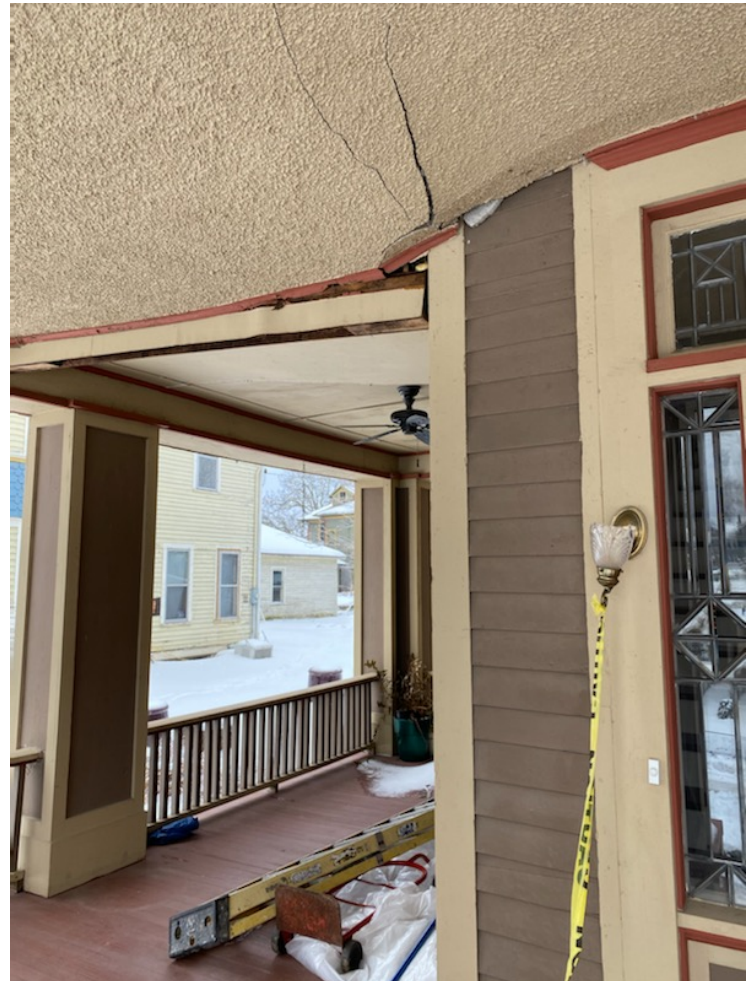
Stucco Ceiling to be Repaired and Painted to Match Existing Color & Material
