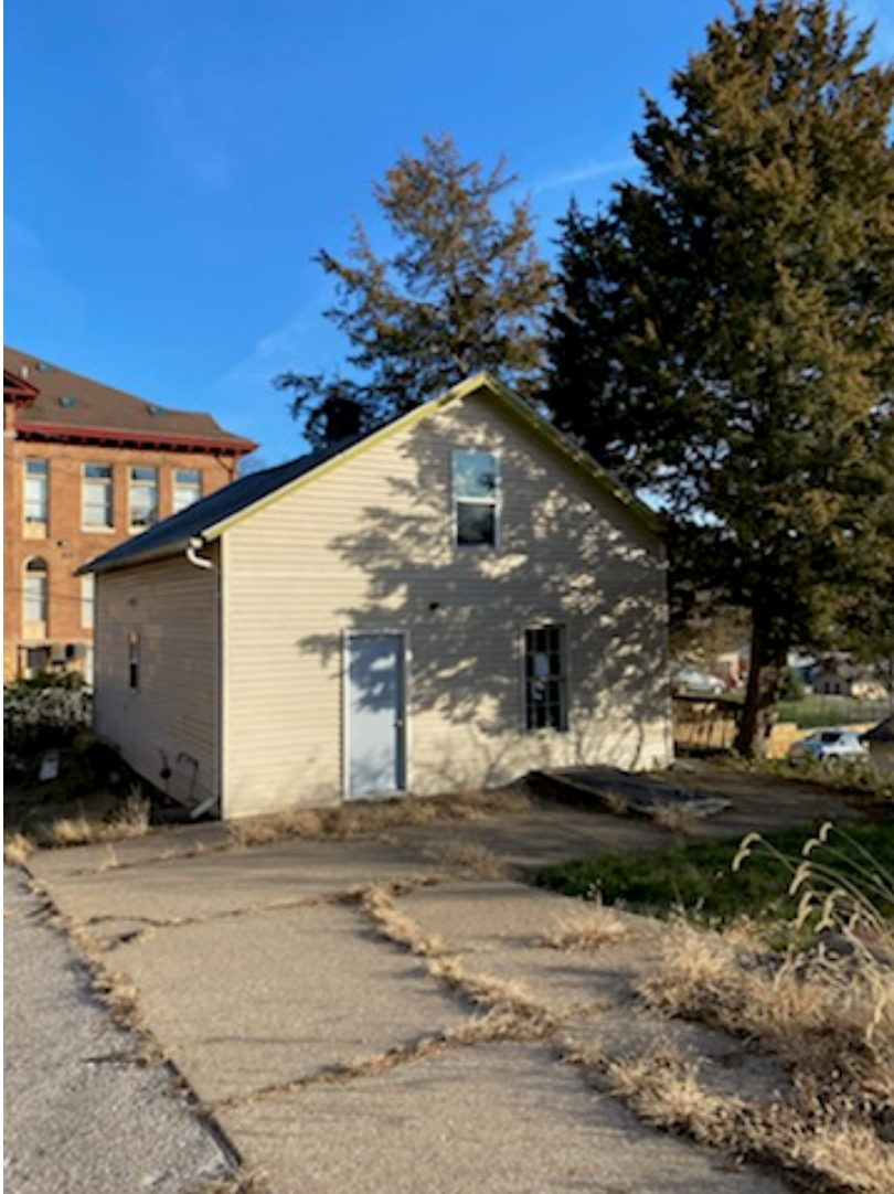
West Elevation-View From Backyard
