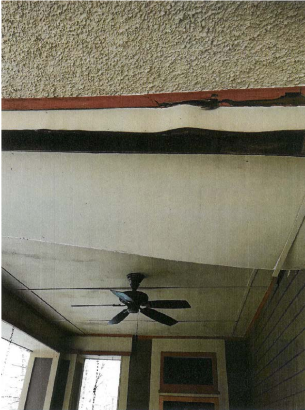
Northwest Section of Porch
