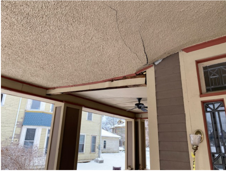
Structural Beam on Porch Ceiling to be Replaced
