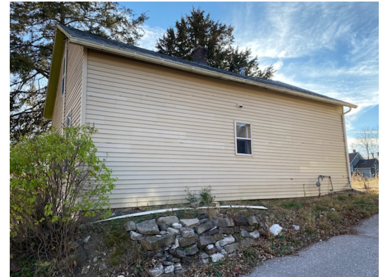
North Elevation-View From Alley
