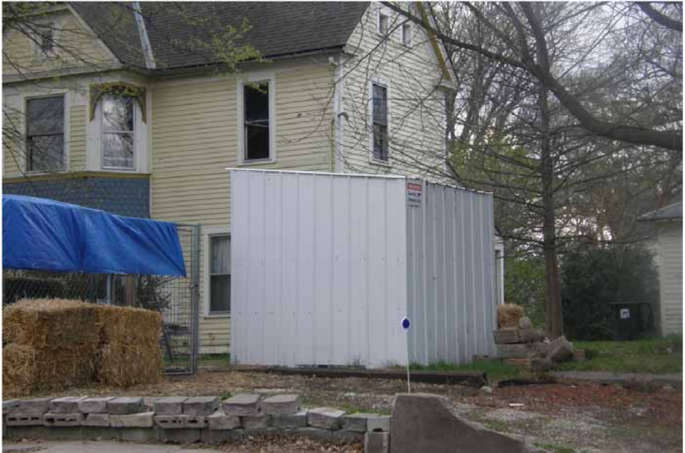
Photograph 82-00681-004 - House, looking southwest (April 2015)
