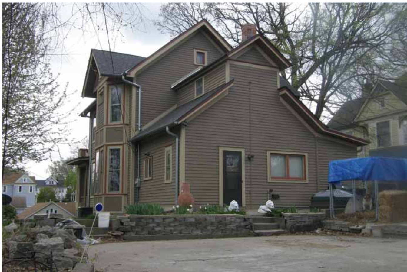
Photograph 82-00681-003 - House, looking southwest (April 2015)
