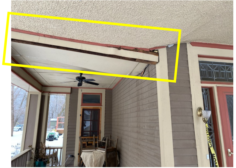
Structural Beam on Porch Ceiling to be Replaced
