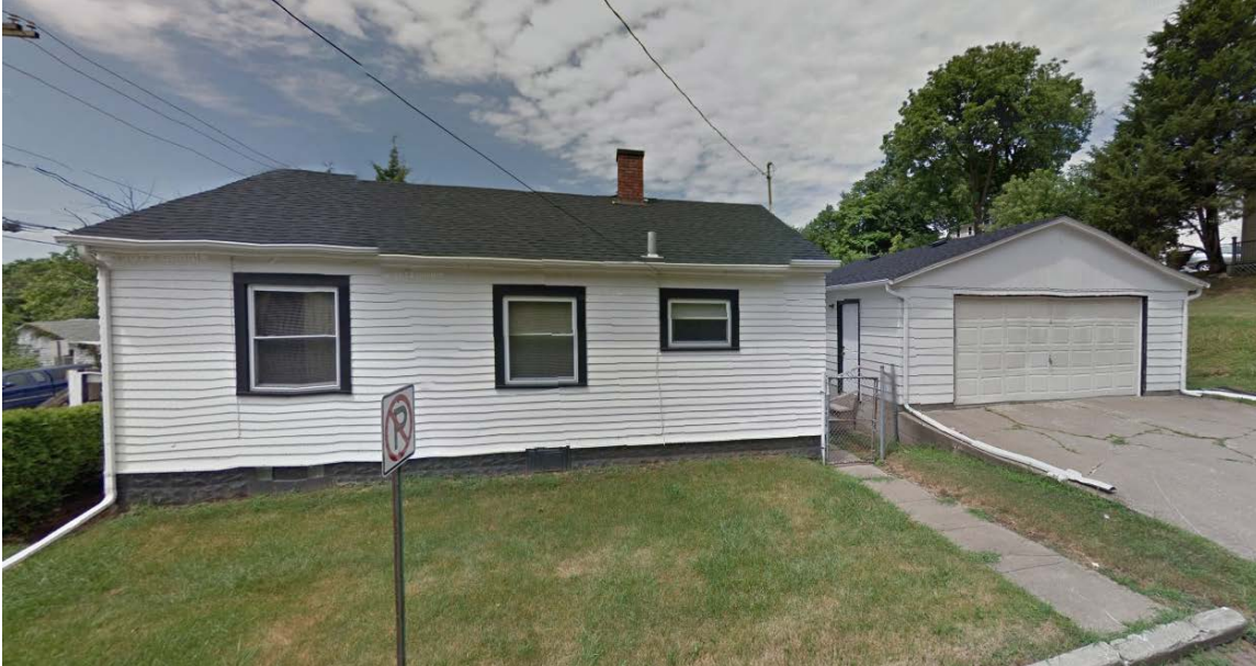
2122 East 12 th Street Property Directly South – View from Christie Street
