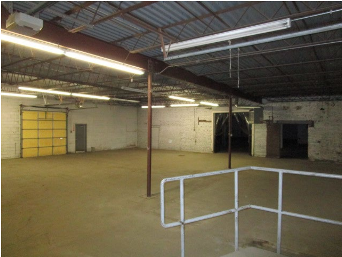
Photo #24. Addition looking NE, shot 01-08-19.
