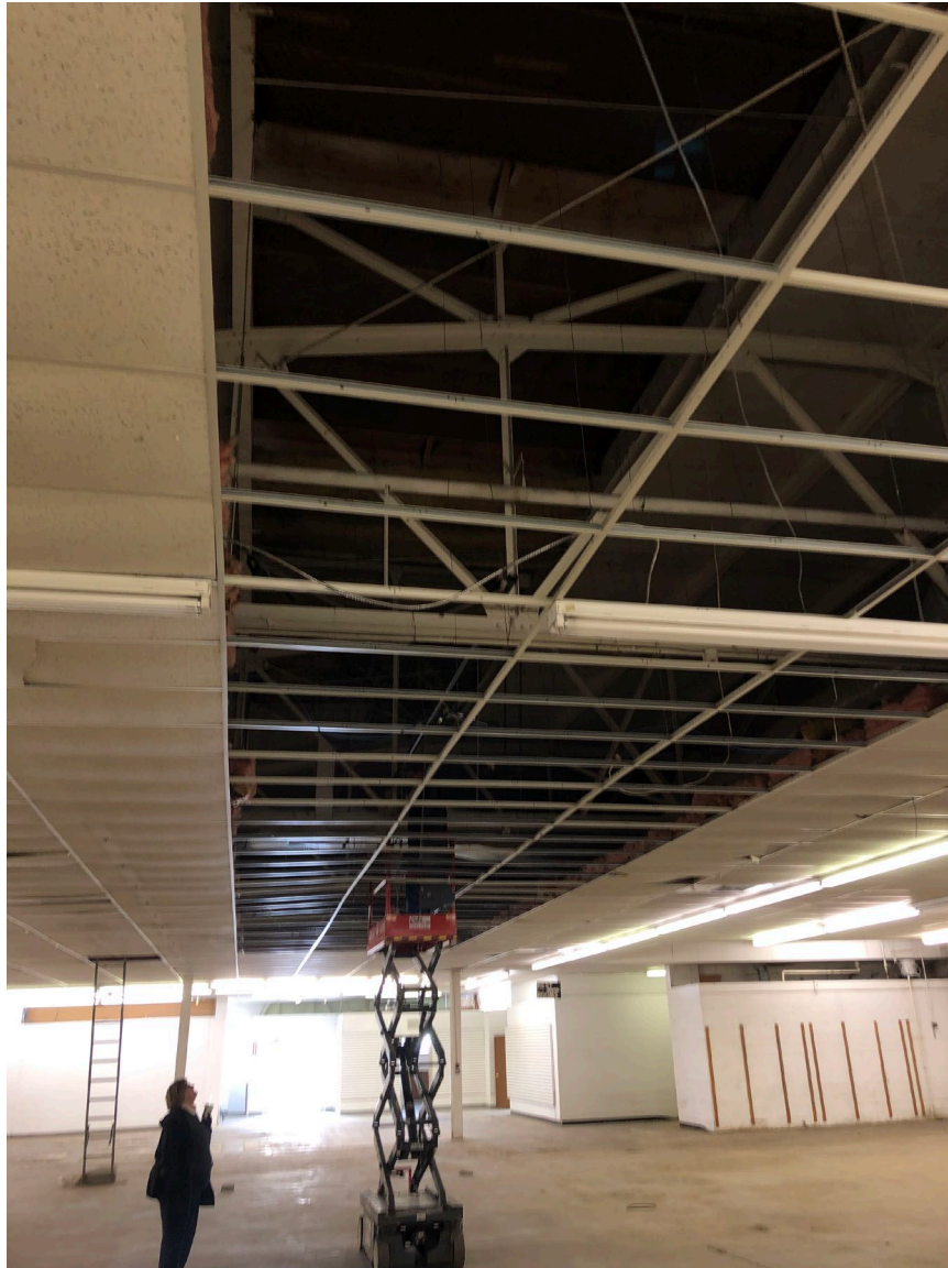
Photo #21. Roof trusses exposed looking N, shot 01-08-19.
