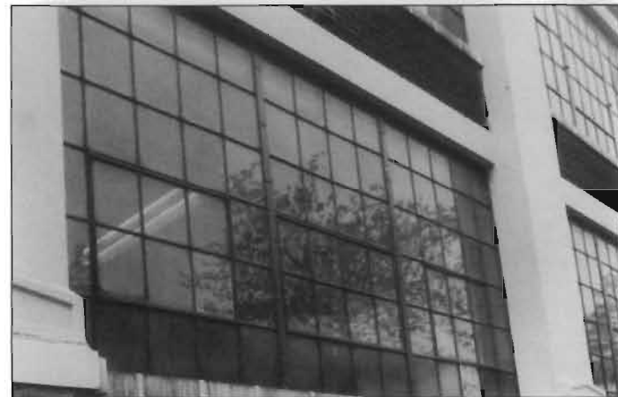
The steel pivot windows in this historic manufacturing building were replaced with new windows which matched the multi-lighted originals.
