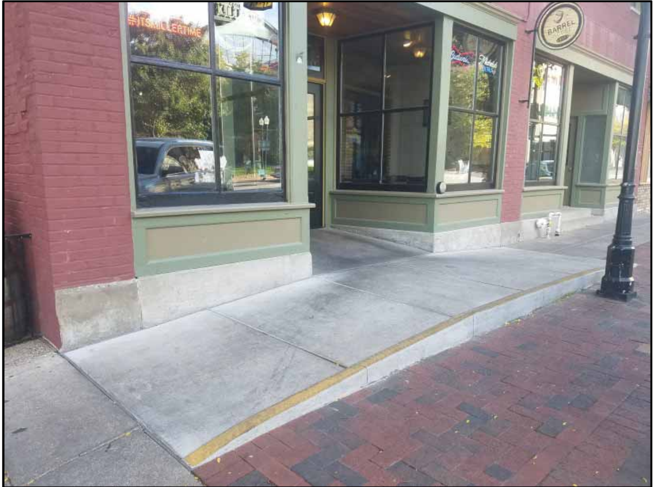
Figure 17. Accessible entrance to 211 East 2 nd Street
