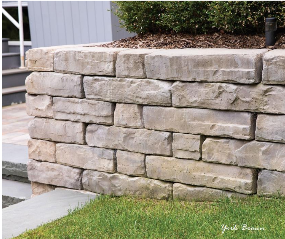
Kodah Block Retaining Wall
