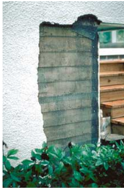
Preparation for stucco repair.
