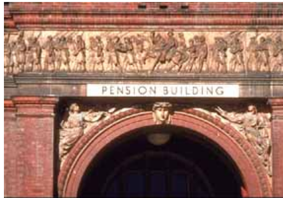
1880s brick building with terra-cotta trim.
