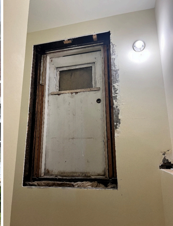
Interior photo of window on back staircase landing
