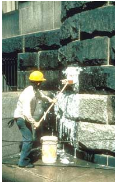
Chemical cleaning to remove dirt from granite.
