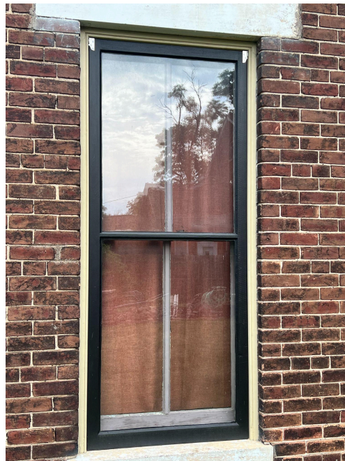
Wood-framed storm window in kitchen to be placed over replacement window
