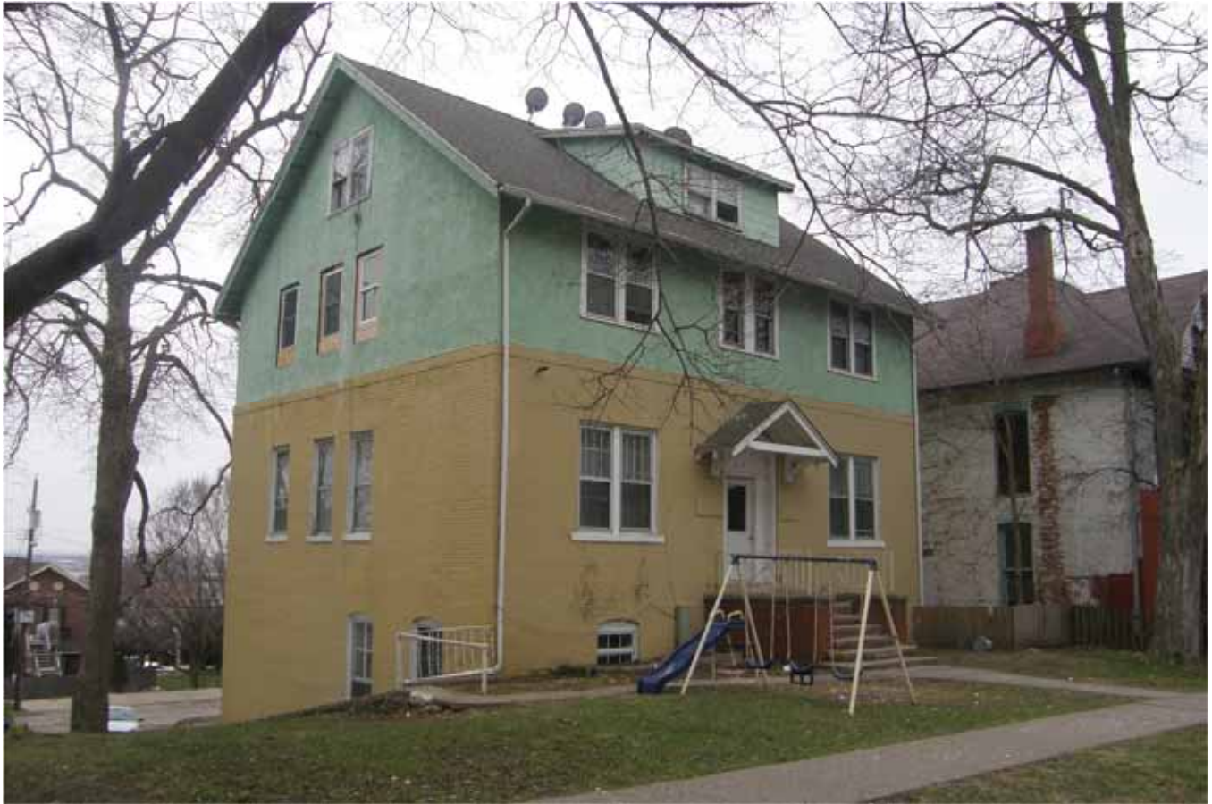
Photograph 82-00552-001 - House, looking southwest (April 2015)
