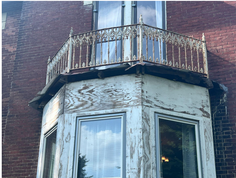
B. Flashing, membrane, and railing above bay window
