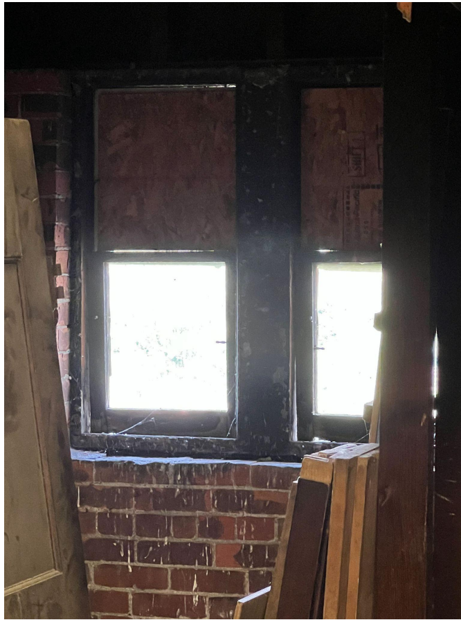
Interior view of east window in center of home
