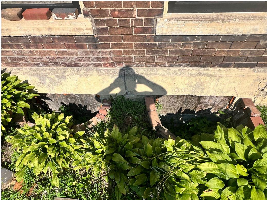
H. Close up exterior view of basement windows on west side of home
