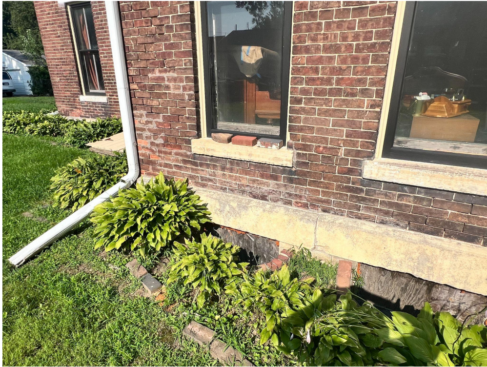
G. Exterior view of basement windows on west side of home
