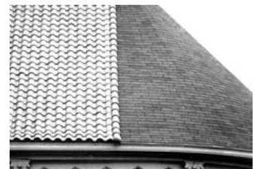
Asphalt shingles are an incompatible replacement substitute for the original Spanish clay tiles. Photo: NPS files.
