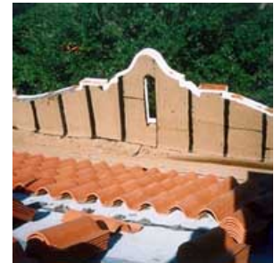
Projections on the underside of these replacement Spanish clay tiles help them adhere to the cement mortar on the roof sheathing. Photo: NPS files.
