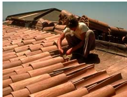
These tapered barrel clay tiles were accurately reproduced from archeological materials found on site. Photo: NPS files.
