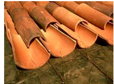
A special system consisting of brass or copper wires is used to attach these tapered barrel roof tiles. Photo: NPS files.
