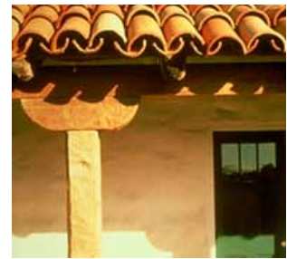
Historic clay tile roof. Photo: NPS files.
