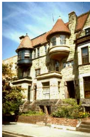
Clay tile was a popular roofing material for residential structures during the Romanesque Revival period. Photo: NPS files.
