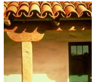
Historic clay tile roof. Photo: NPS files.
