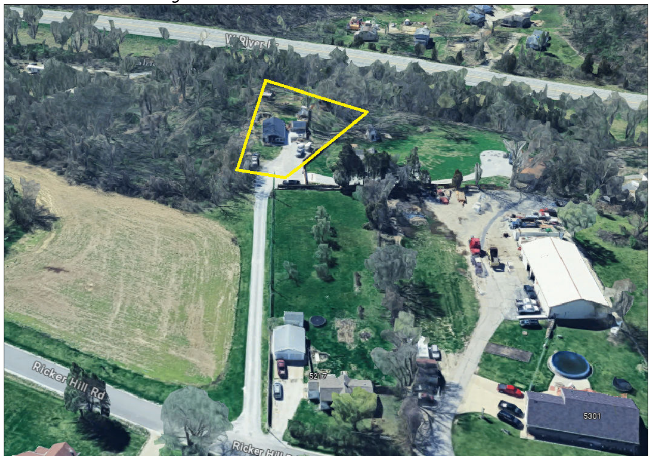
Aerial Site Photo: Facing South from Rickerhill RD
